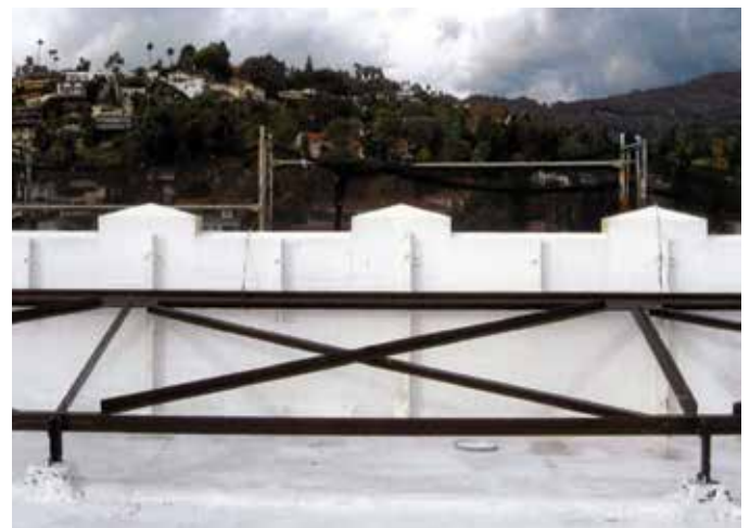
Figure 20. Bracing parapet walls, as illustrated in the typical detail drawing on the left, and as installed in the image on the right, helps avoid hazards from falling debris.
