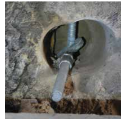
Figure 26. Eye bolts used to anchor the floor to the wall.
