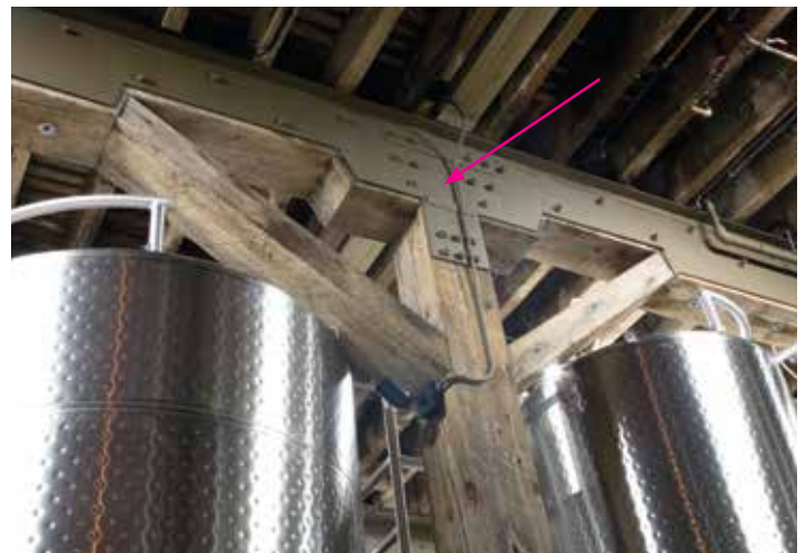
Figures 17 and 18. Careful placement of the new structural reinforcement, painted to match the surrounding building elements, if left exposed, minimizes its visual impact. New added structural elements may be left exposed when their visibility does not impair the historic character of the building. Figure 17 (left). Photo: Jason Hagin. Figure 18 (right). Photo: Architectural Resources Group.
