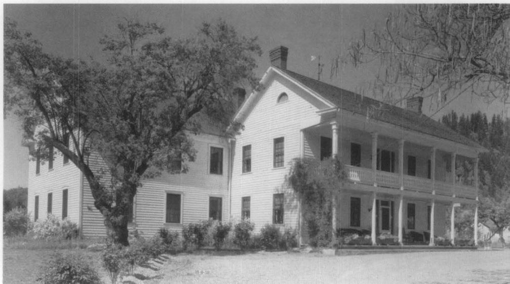
Figure 14. The treatment approach selected for a building usually is determined by the intended use of a property, funding prospects, and the findings of an investigation. The Wolf Creek Inn, operated by the Oregon Parks and Recreation Department, is among the most intact and oldest active travelers' inns in Oregon. The historic structure report outlined a rehabilitation treatment which included such work recommendations as repairs to specific historic fabric, landscape restoration and site improvements, and upgrading of the building's mechanical and electrical systems. Photo: Historic American Building Survey, 1934.
