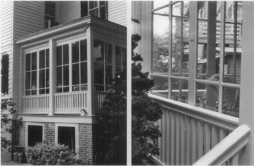
Figure 12. This old porch enclosure, located on the back side of a house, has acquired significance over time and is remarkable both in the appropriateness of its detailing for use by others today, as well as its high degree of maintenance. The enclosure is set behind the columns; the balustrade has been retained; and the light divisions and the size of the glass panes echo that of the windows above. Within each bay there are two well-crafted, inward swinging doors, providing for greater seasonal use of the porch. Photos: Charles Fisher.
