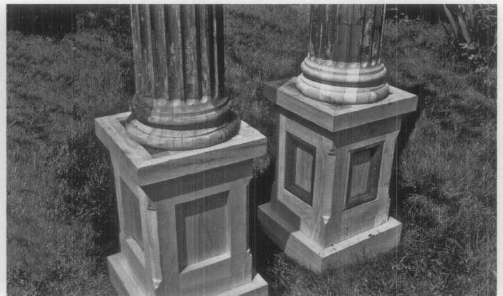
Figure 10. This nineteenth century porch column is made of wood staves, similar to the way a wood barrel is put together. After replacing the torus and making dutchman repairs to the apophyge along the base, the column and pedestal are ready to be reinstalled on the porch. Photos: NPS files.
