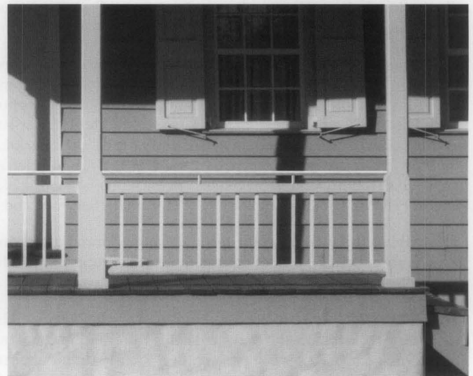
Figure 19. Historic porches generally have railings that measure 28 to 30 inches in height from the floor. When additional height is necessary for safety, a simple rail, added for illustration purposes in this photograph, can usually be installed above the historic railing. Not only does this treatment allow retention of the historic balustrade, but it also has a minimum impact to the appearance of the porch. Photo: Charles Fisher.
