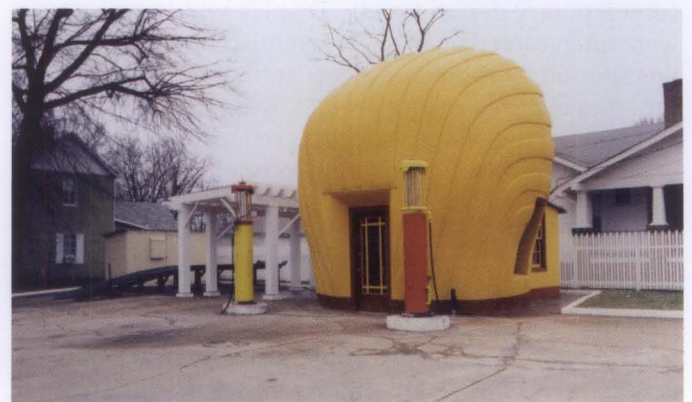
Figure 5. This 1936 Shell station in Winston-Salem, NC, is an example of a programmatic design, meant to attract attention and stick in the customer's mind. It was recently rehabilitated to serve as a field office for Preservation North Carolina. Photo: Preservation North Carolina.
