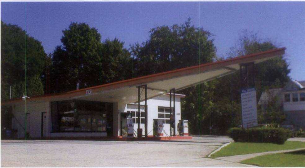
Figure 8. This former Phillips 66 gas station in Burlington, VT, sports a quintessential stylized box design. Its space age canopy is visible from far down the road. Photo: Devin A. Colman.
