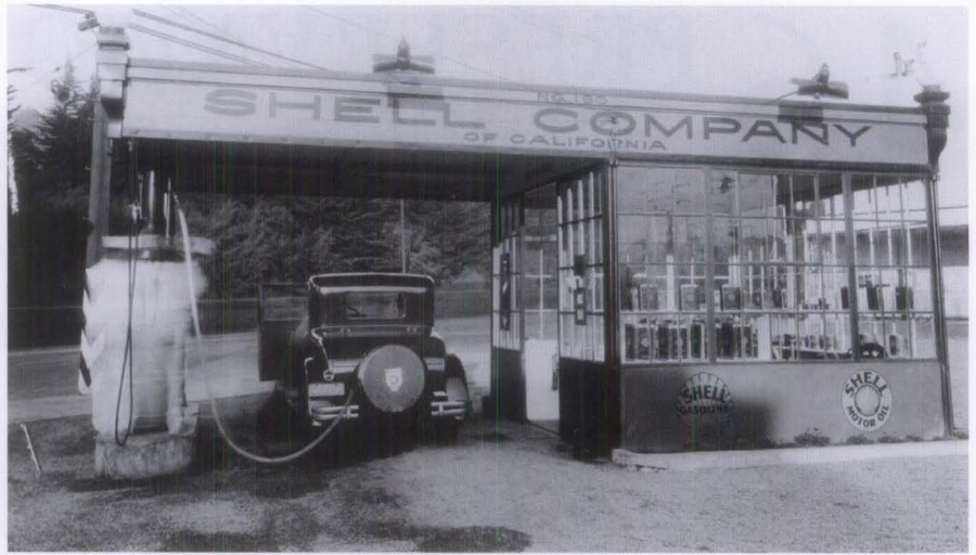
Figure 3. This shed-type station with its prefabricated steel panels, pump island, and canopy prefigured many later gas station designs. Photo: American Petroleum Institute Photograph and Film Collection, Archives Center, National Museum of American History, Smithsonian Institution.
