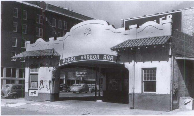
Figure 12. Gas stations have a long history of reuse (and abandonment and reuse again). By 1942 this gas station in Tulsa, OK, was already being reused as a bar. At one time the front island shed (on the left) functioned as a locksmith's shop but was vacant at the time of the photo. Photo: Library of Congress, Prints and Photographic Division, LC-USW3-9523-D.
