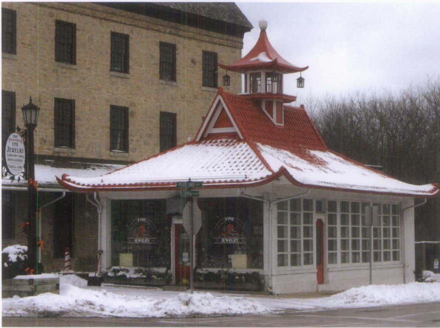
Figure 9. The dominant feature of this former gas station (1929) in Cedarburg, WI, is its pagoda-style metal tile roof (complete with upturned eaves and Japanese lanterns suspended from the cupola). The building currently functions as a jewelry store. Photo: Kenneth M. Itle, Wiss, Janney, Elstner Associates, Inc.
