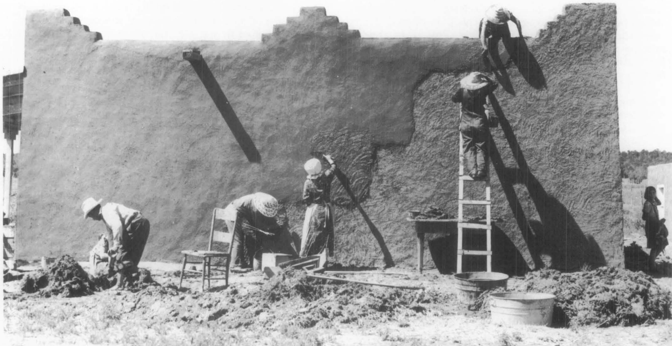
Renewing the Surface Coating. Traditionally, adobe surface coatings that protected the fragile adobe building fabric were renewed every few years. Recently however, high labor costs have made this a relatively expensive process. Women are seen here recoating an adobe wall with mud plaster mixed with straw at Chamisal, New Mexico. (Photo by Russell Lee, Farm Security Administration Collection, Library of Congress)
