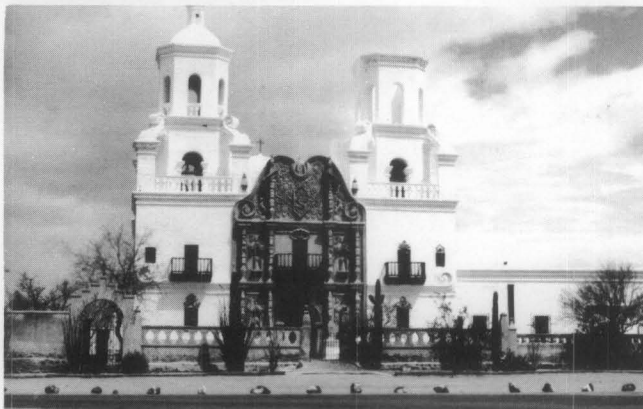
SAN XAVIER DEL BAC, TUCSON VICINITY, ARIZONA. Built entirely of adobe construction (1783–1797), this is one of the finest Spanish Colonial churches in the United States, having an elaborate frontispiece of molded, carved, and painted brick imitating stone. (National Park Service)
