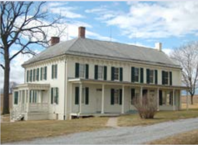
Figure D. Tall lightning rods once again stand out on the Mumma House. These reproduction rods along with retention of the historic down conductors have been incorporated into the modern lightning protection system that was installed. Much smaller, contemporary air terminals located on the roof are barely discernible from below. Photo by author.
