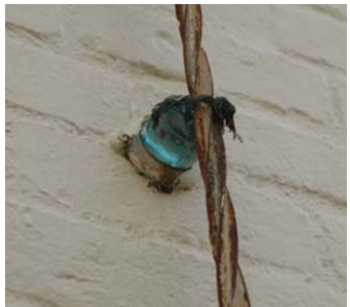
Figure 17. Glass insulators were attached to a structure in a variety of ways using metal rings, staples, wire, or similar fasteners. Where old insulators are damaged and no longer functional, they can be replaced with appropriate metal fasteners. Photo by author.
