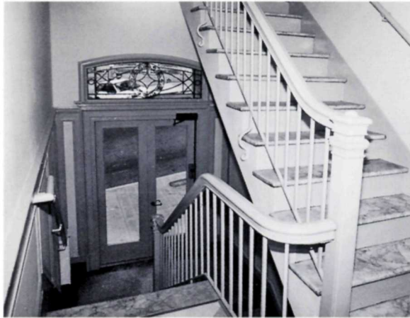
A rehabilitated stairway in the Pacific Hotel.
