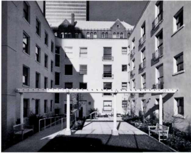
The rehabilitated courtyard, fully accessible from the lobby.
