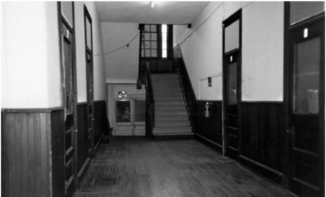
Shelly School classrooms (top) and halls (above) prior to rehabilitation; historic features and finishes were preserved in the rehabilitation.
