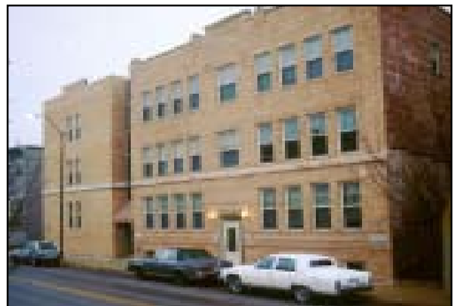
The slight recess at the intersection of the addition (left) and the historic facade (right) allows the visual mass of the original building to remain unchanged.
