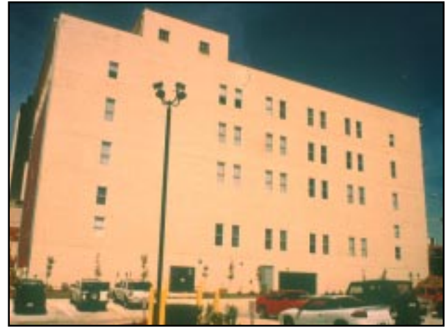
Simple, compatible openings were cut into this blank, non-significant secondary elevation when the building was rehabilitated for apartments.
