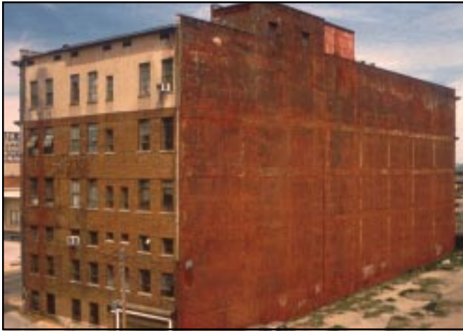
Simple, compatible openings were cut into this blank, non-significant secondary elevation when the building was rehabilitated for apartments.
