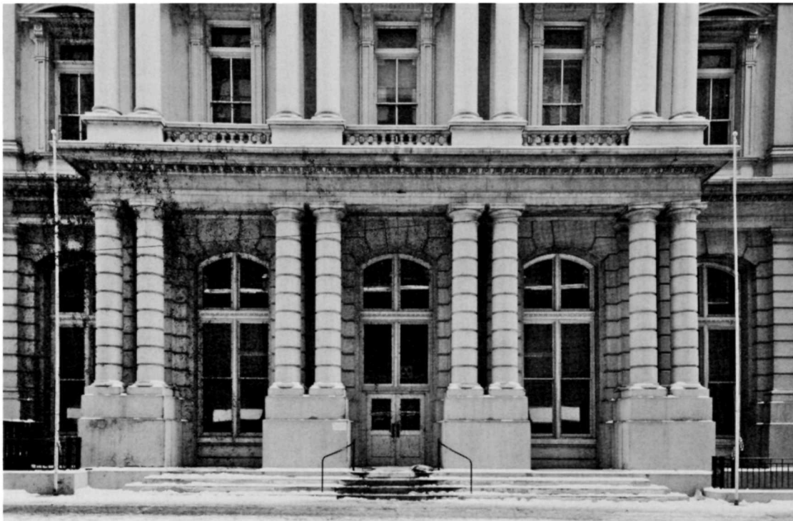
Ninth Street pavilion, showing rusticated columns, pilasters, and walls at the first floor level. (Photo by Paul Piaget, 1965.)
