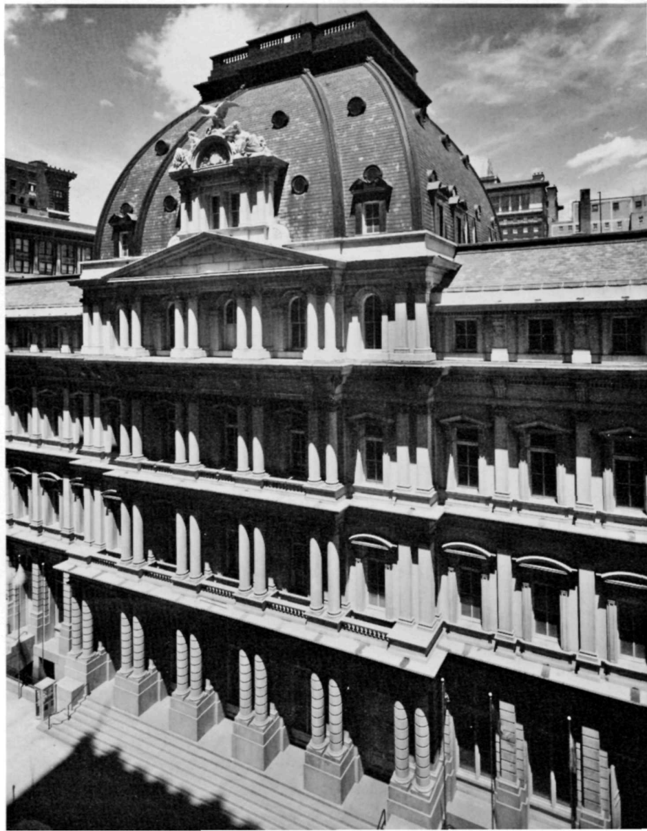
Olive Street entrance pavilion of Old Post Office. Coupled columns, segmental and triangular pediments over windows, and cornices acting as belt courses are all reminiscent of the State, War, and Navy Building. (Courtesy Arteaga Photos.)
