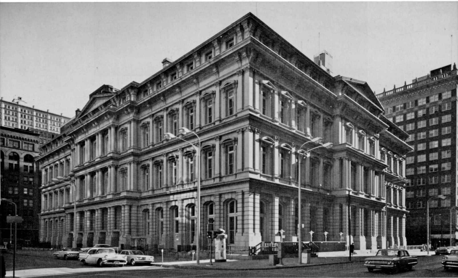
This view of the Ninth Street and Locust Street (rear) facades clearly shows the superimposition of classical orders. (Photo by Paul Piaget, 1965.)
