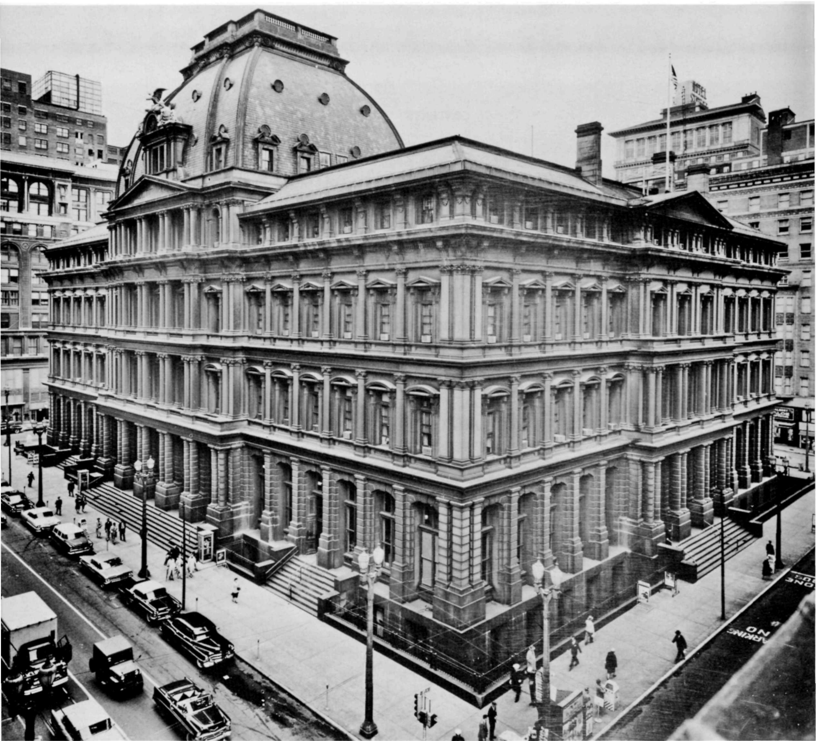
General view of the Old Post Office. Olive Street facade is to the left, and the Eighth Street facade to the right. The wall surfaces are highly articulated with recessed window and door openings divided by pilasters and columns. The depressed areaway or "moat" can be seen between the building and the sidewalks. (Photo by Paul Piaget, 1965.)
