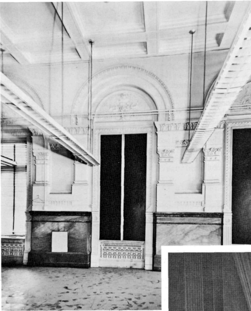
Large chamber. Finish includes marble wainscoat, cast-iron mouldings and ventilation grilles, and plaster ornamentation. Window at center has sheet iron shutters closed.
