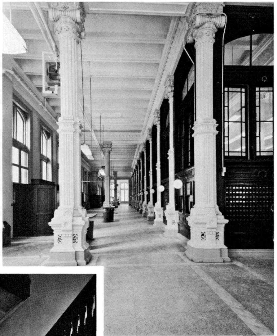
First floor Post Office. Outlets for circulating hot air heating systems are in the column bases.
