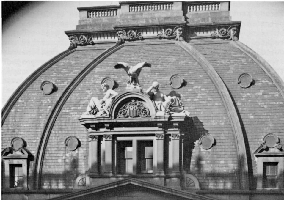
Near view of the mansard dome on the Olive Street facade which was originally topped by an ornamental belvedere. (Photo by Paul Piaget, 1965.)
