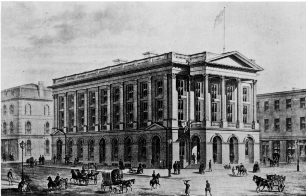
U.S. Court House and Post Office in Portland, Maine. Built 1867-1873. One of the numerous smaller government buildings designed by Mullett and a fine example of his work in the Classic Revival style, this structure was demolished in 1965. (Photo copy of 1868 perspective by Von Koerber.)
