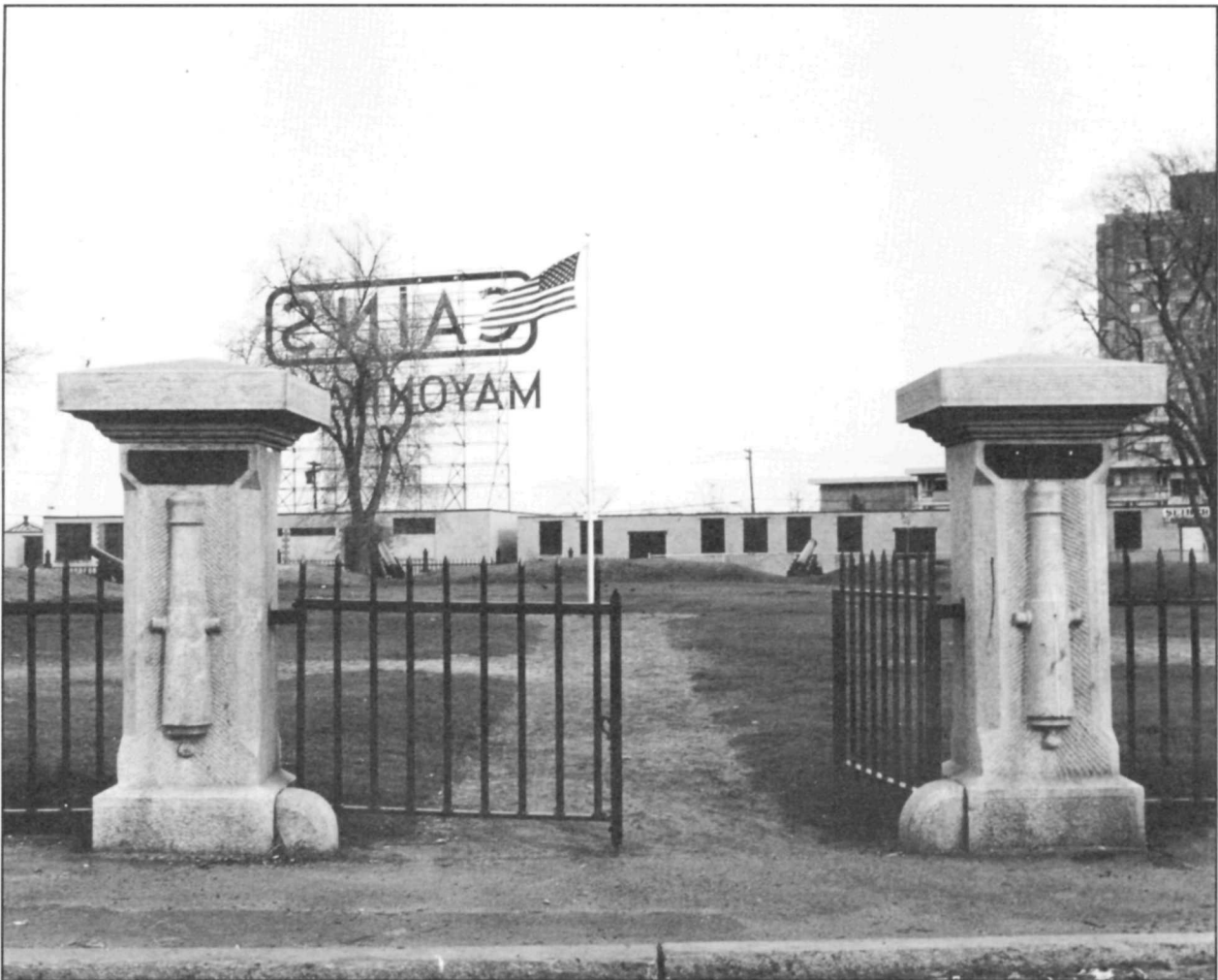
Granite, although one of the harder building stones, still lends itself to carving as illustrated in the carved cannons on these entry pylons at Fort Washington, 1858, Cambridge, Massachusetts. John R. Hall, architect. Photo: Cambridge Historical Commission.
