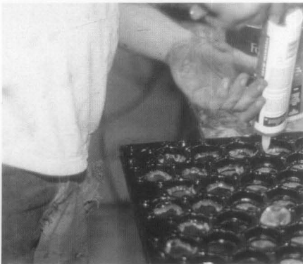
Figure 8. Before the glass lenses were set, a ring of silicone was placed along each flange on the lower edge of the opening. The silicone kept the lens centered in the cavity while a waterproof grout was used as the main sealer.
