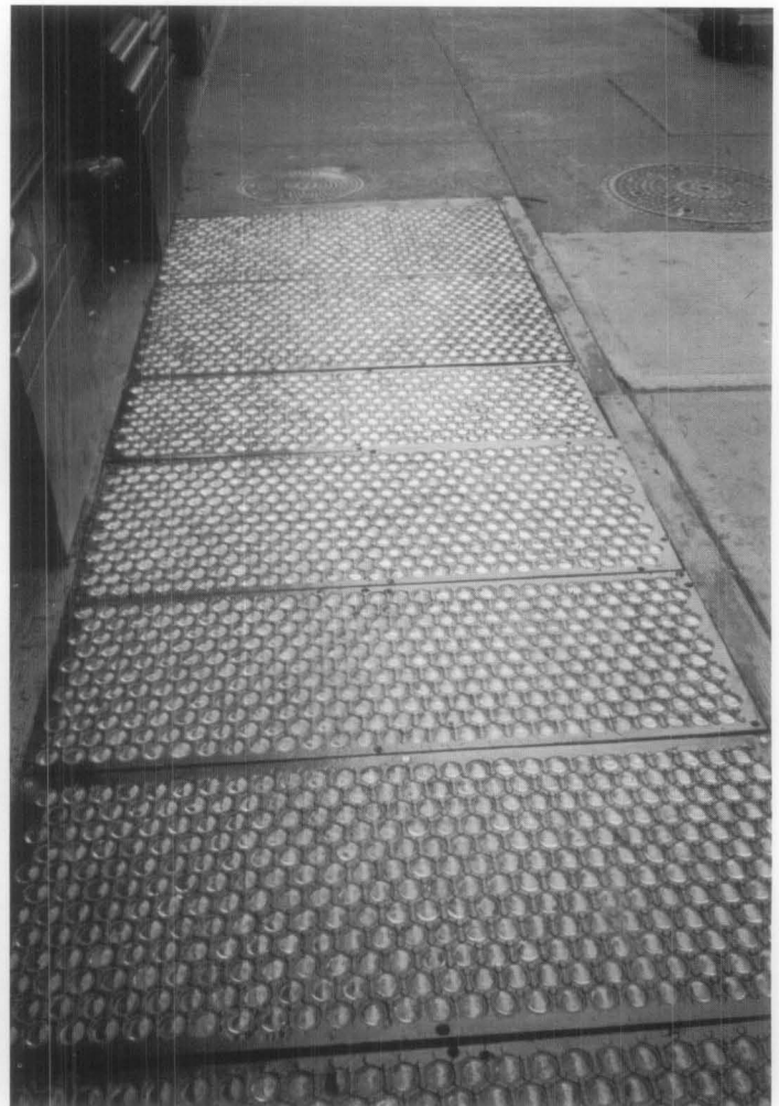
Figure 14. The restored panels after work was completed.
