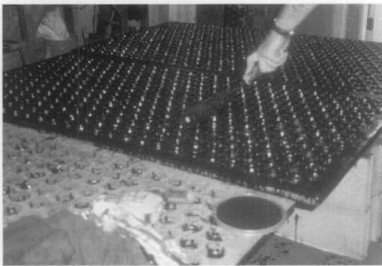
Figure 7. Cleaned and repaired panels were painted with two coats of oil-based metal primer and three alkyd gloss enamel top coats.
