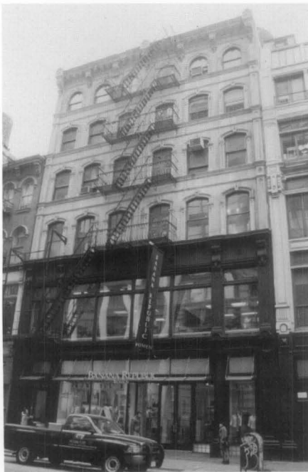
Figure 1. A cast-iron storefront was added to 552-554 Broadway in 1897. The storefront included a fifty-four foot long assembly of cast-iron vault lights set in the sidewalk. Glass lenses in the panels allowed light to enter the basement area, increasing rentable space for the building owner.
