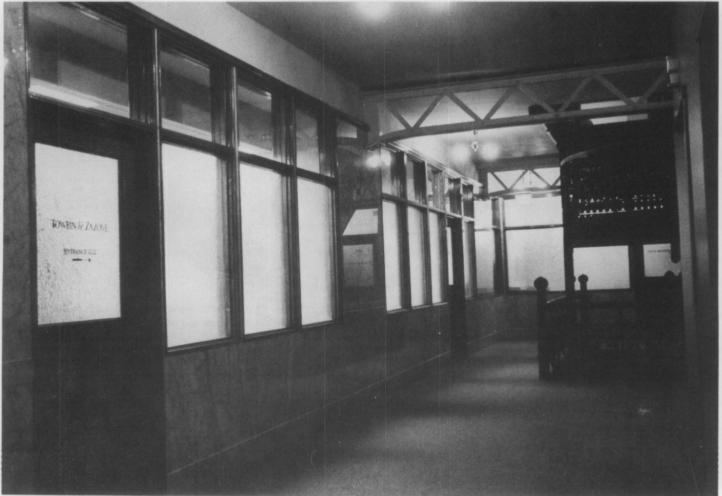
Figure 10. Rehabilitated corridor showing marble wainscot, oak and feather-chipped glass corridor partitions, full ceiling height and open ornamental stairs. Photo: Ron Gordon
