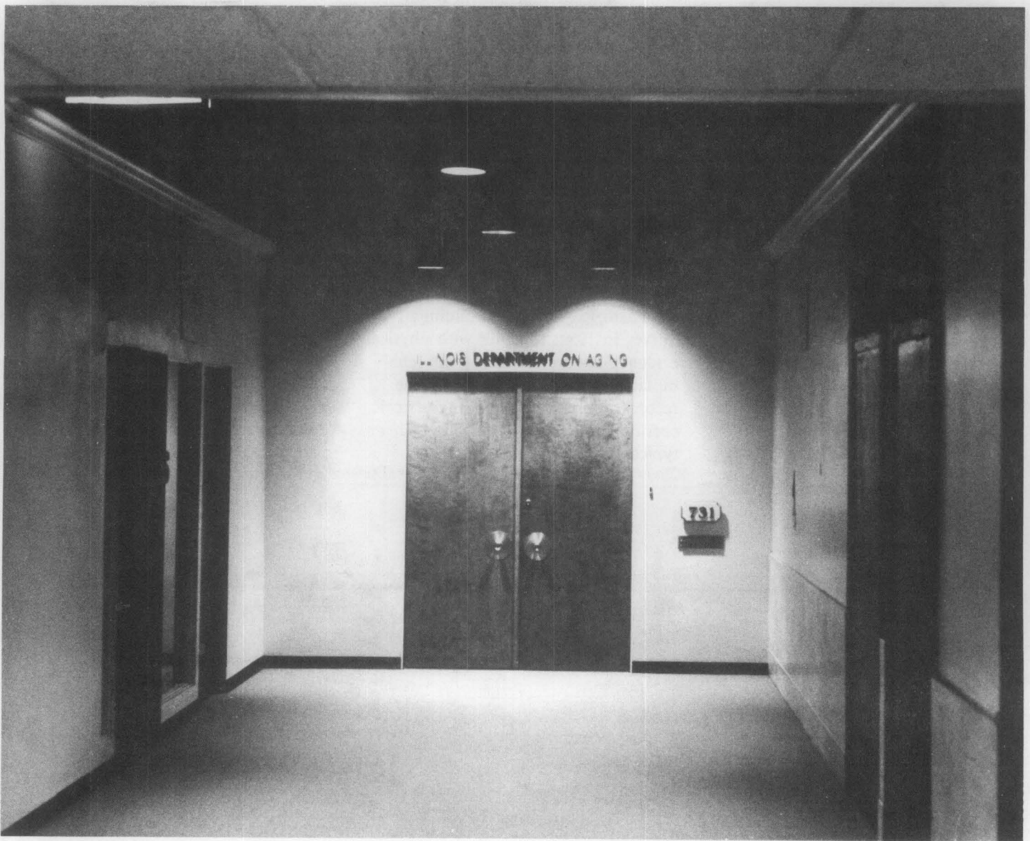
Figure 2. Typical condition of public corridors prior to rehabilitation. Glass and oak corridor partitions and much of the marble wainscot was either removed or covered. Ceilings were suspended and sections of the corridor plan were shortened or removed. Photo: William S. Donnell
