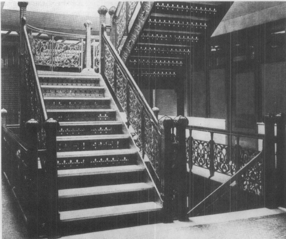
Figure 8. Burnham and Root's aluminum and bronze plated cast-iron stair remains the most notable architectural feature in the north half of the building. Minor repair work and a few missing elements have been replaced with cast aluminum. Favorable building codes allowed the open design.
