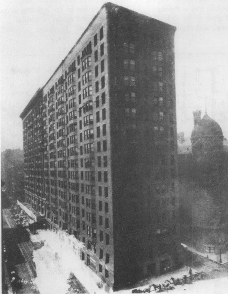
The Monadnock Building Chicago, Illinois
