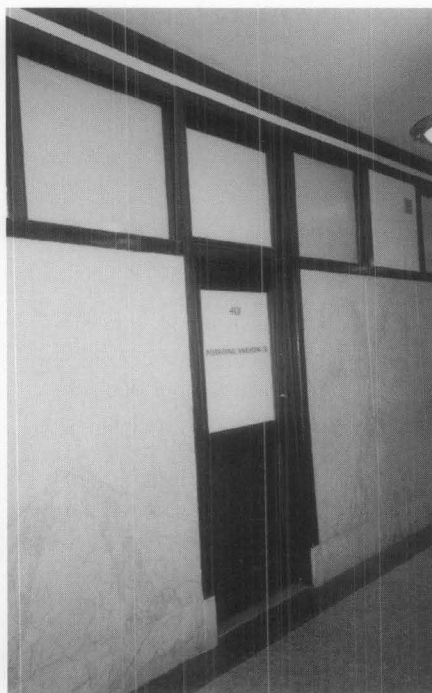
Figure 10. Completed Fisher building corridor with back painted door and tripartite transom. Photo: National Park Service File.
