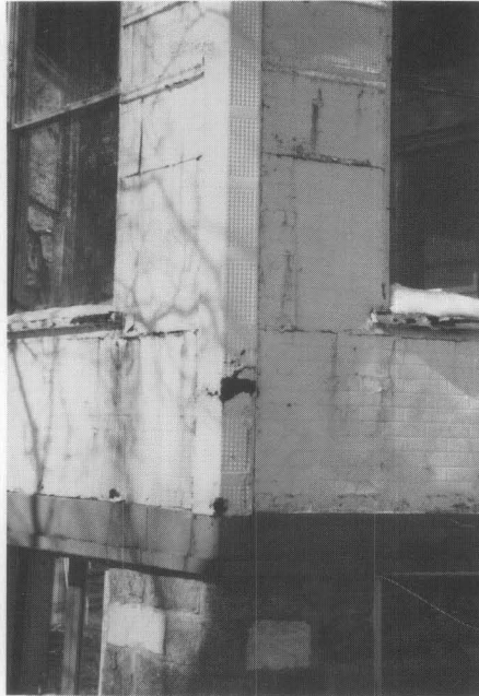
4. Rust stains indicate where corrosion, caused by water infiltration, are breaking through the metal from the rear. Rust and separation are also evident at seams between sheets of stamped metal. Inspection determined that nearly 90% of the stamped metal siding had to be replaced. Photo: Richard Hiler.
