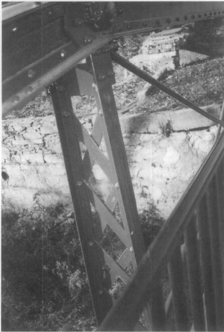
Figure 10. The new lattice girders are shown as installed on the bridge. Photo: Joseph P. Saldibar, III.
