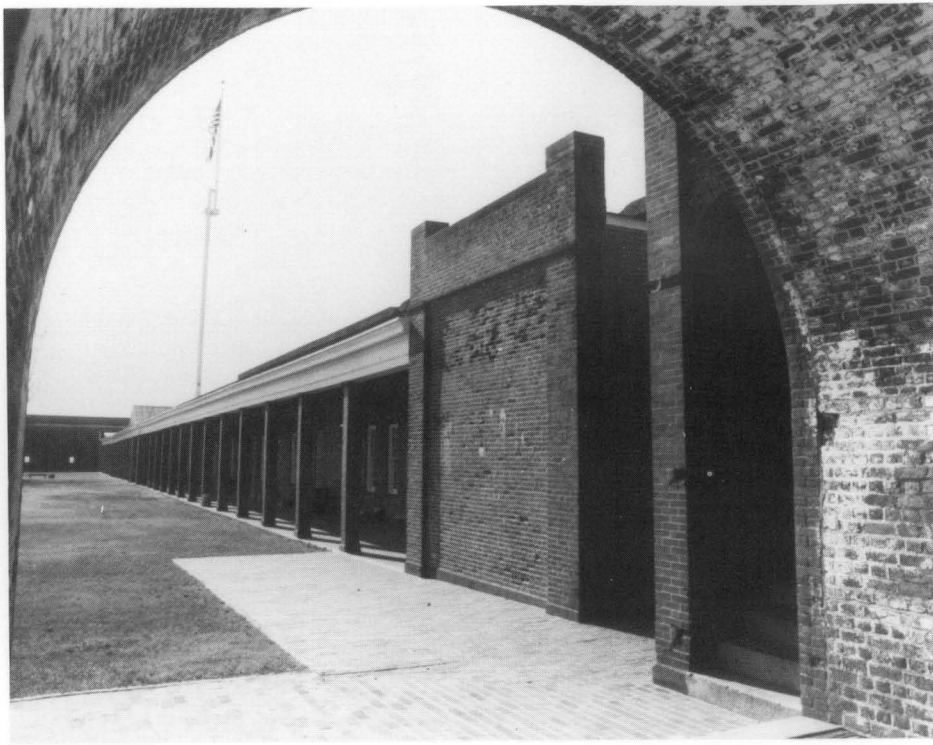
Figure 2. View from one of the open casemates, looking across a portion of the parade ground. The piazza provides a covered access to the enclosed casemates which flank the sally port. It was one of these enclosed casemates (each has a door and one or two windows) that was selected to house the museum object storage facility.
