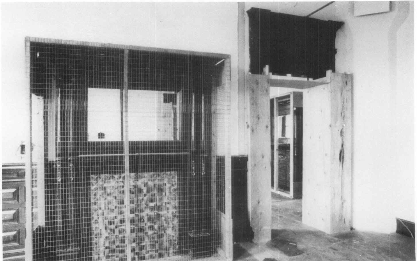
Figure 6. A self-supporting impact cage utilizing wood and wire mesh protects the fireplace. In this project, the long construction process required bidders to have visible access to features such as the fireplace. The wire mesh also facilitated monitoring during the lengthy construction. Photo and drawing: Ford Farewell Mills and Gatsch Architects.
