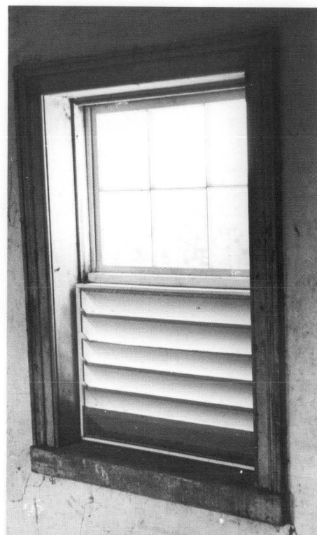
Figure 5. Screening was attached to the back side of the louvers to prevent the recurrence of insect, bird, and rodent infestation. Photo: Charles Fisher
