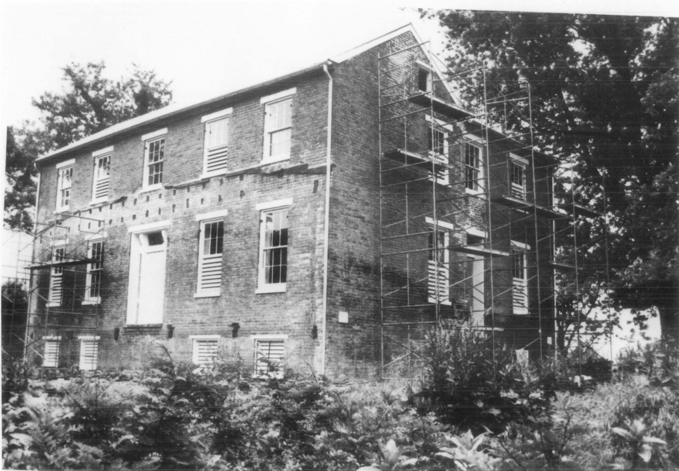
Figure 6. The window louvers installed in the Worthington House have proven effective over the past two years in providing the necessary ventilation for the building. Photo: Tom Vitanza.
