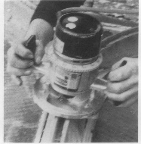
Figure 4. Once the old paint had been carefully removed, grooves were cut in the mullions using an electric router fitted with special guide rollers.
