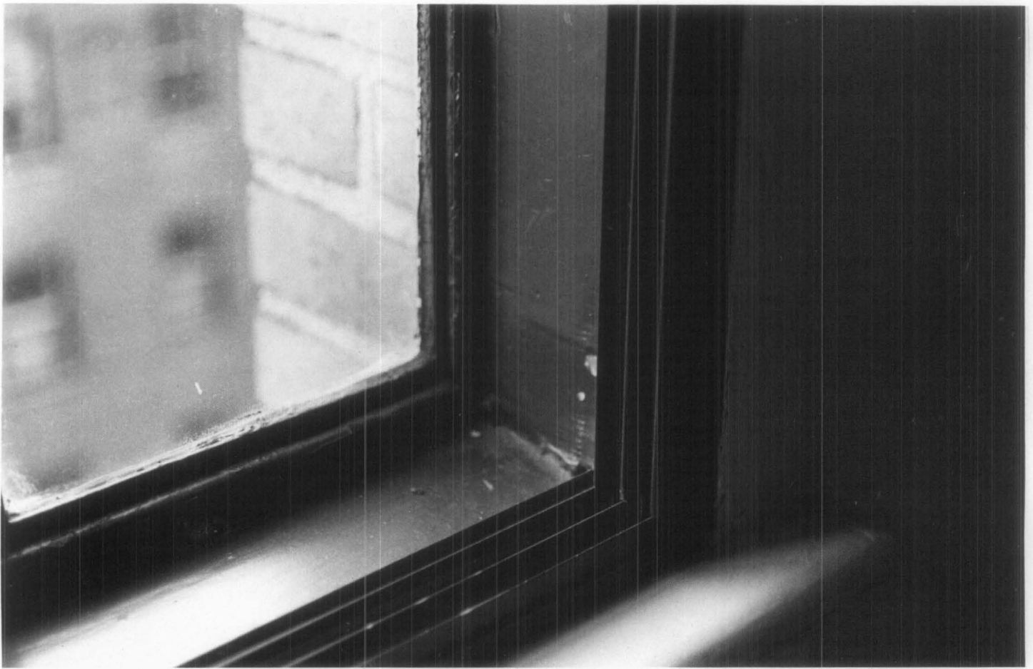
Figure 6. The subframe had to be squared off when installed in each window opening to prevent racking of the sliding panels. Photo: Christina Henry.
