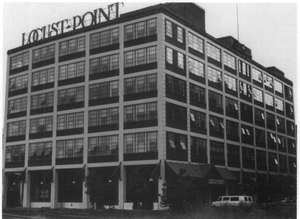
Figure 13. Lippincott Press Building (now Locust Point) after repair of the multi-light steel windows. Photo: Robert Powers.
