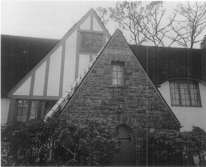
Figure 1. Steel casement windows were placed in various configurations throughout the house. Grouped windows open in opposite directions from each other, assuring that breezes can be captured, and a sash opened during rainy weather, regardless of the wind direction.
