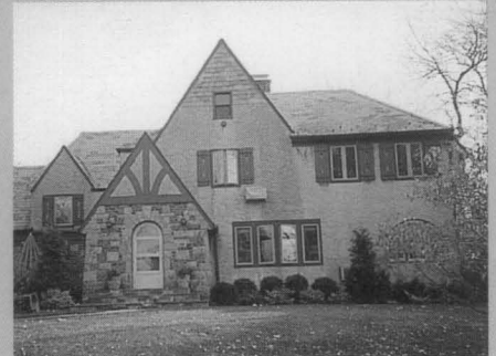
Inappropriate replacement windows dramatically affect the appearance of a historic home that once featured steel casement windows.
