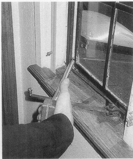
Figure 6. Pull bars were used to realign the sash from the inside. These custom made tools were especially useful on single sash units where the worker was unable to reach through an adjacent opening to apply pressure from the outside.
