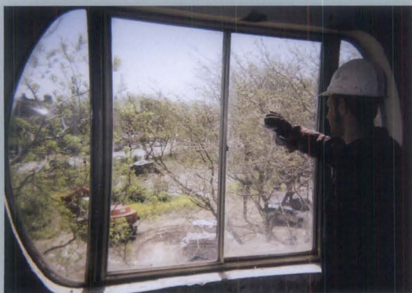
Figure f. Repair and replacement work was done from the inside to lessen the risk of damage to the outside finish. (Photo: Holsten Real Estate Development Corp.)
