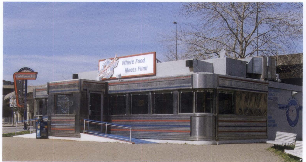
Figure 10. The shine and luster of an aluminum window with an original mill finish was a perfect compliment to the stainless steel exteriors found on 1940s/1950s diners. The Hollywood Diner is an authentic Mountain View Diner built in 1954. It first operated in Westbury, New York and was later moved to Baltimore, Maryland. In the 1980s it was the location site for several Barry Levinson's films including "Diner." Most of the original windows remain in this building.
