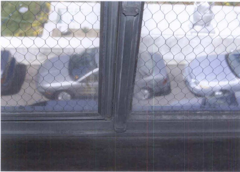
Figure 13. As early as the 1930s, companies primarily making aluminum windows often offered an option for an aluminum storm window, usually on the exterior. The left-hand photograph shows an early interior storm window piggybacked onto the primary window frame at the Folger Shakespeare Library (glass pane on the left). The photograph of the same window, from the outside, shows no indication of an interior storm.
