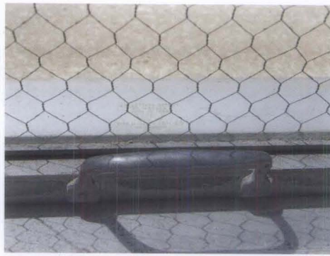
Figure 14. Hardware for early aluminum windows came in a variety of materials including steel, bronze, and nickel. Specialty hardware manufacturers can easily replicate suitable replacements today, matching the originals in both material and finish. The manufacturer's stamp, visible through the glass on the exterior sill of this window at the Folger Shakespeare Library in Washington DC, identifies Wm. H. Jackson Company of New York as the maker and dates the window patent to 1926.
