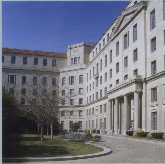
Figure a. In the primary courtyard within the U.S. Department of Justice Building, the aluminum windows emulate the appearance of steel windows with true divided lights. Depending on the floor level and location, the windows differ in size and consist of a varying combination of fixed lights, casements, and a hopper-style unit.
