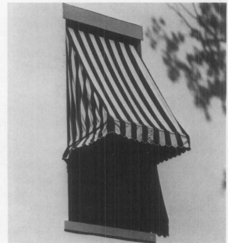
Figure 2. Early photographs were used in determining the appropriate design and size of the new awnings shown in the photograph. Drawing: Courtesy, Shepard Associates, Architects and Planners, Inc.; Photo: Courtesy, Florida Bureau of Historic Preservation.
