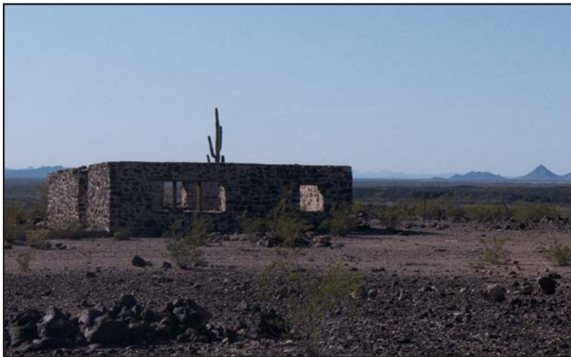
Figure 4.36. This turn-of-the-century building at AZ S:16:9 (ASM), located within the proposed national monument's boundary and affiliated with the South Gila Canal, stands as a memorial to the labors and struggles of efforts to tame the floodwaters of the lower Gila River. (Photograph by Andy Laurenzi.)
