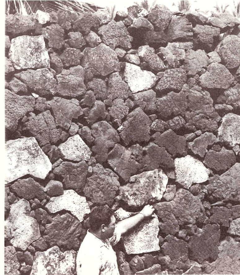
The great wall. A modern Hawaiian inspects the dry masonry of his ancestors.
