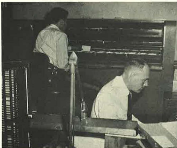
A recent addition—our Diebold elevator file for filing locator cards. (Capacity 250,000 3x5 cards)
