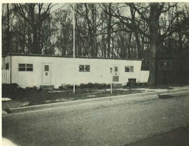
Rock Creek Substation
