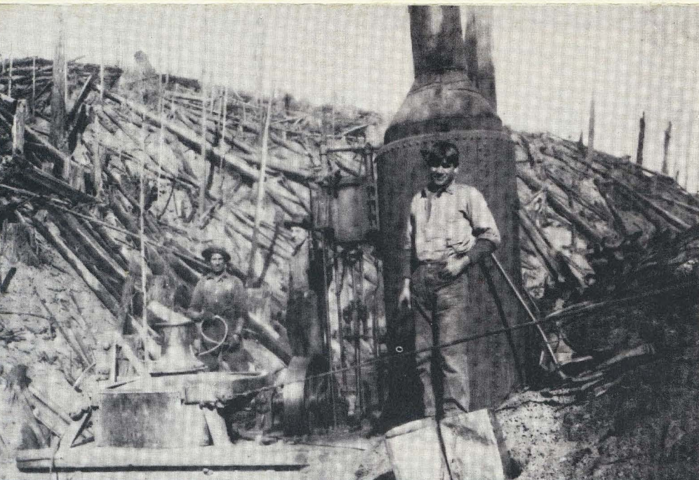
Steam Donkey. Only a few hundred acres of forests in the Redwood Creek watershed were logged before World War II, using such early methods as the steam donkey cable system. The rate of logging was greatly accelerated with the invention of tractors and other modern equipment.
