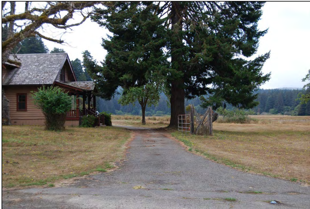
Figure 39. Circulation Features. Driveway to the Boyes House.
