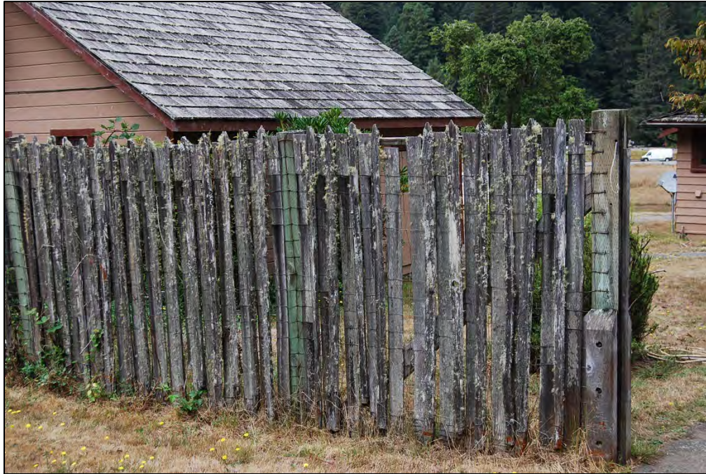
Figure 78. Small-Scale Features. Fence along the backside (east) of the Boyes House.
