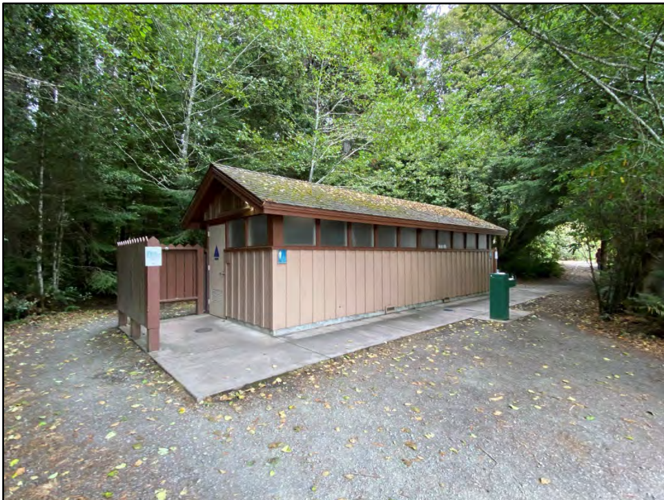
Figure 67. Buildings and Structures. Modern Combination Building adjacent to Visitors Center.
