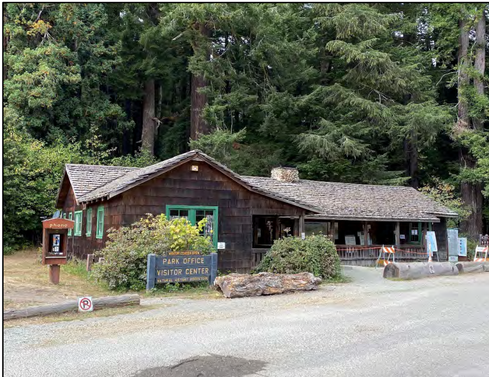
Figure 53. Buildings and Structures. Visitors Center, formerly the CCC-era Park Custodian's Residence (built 1934).
