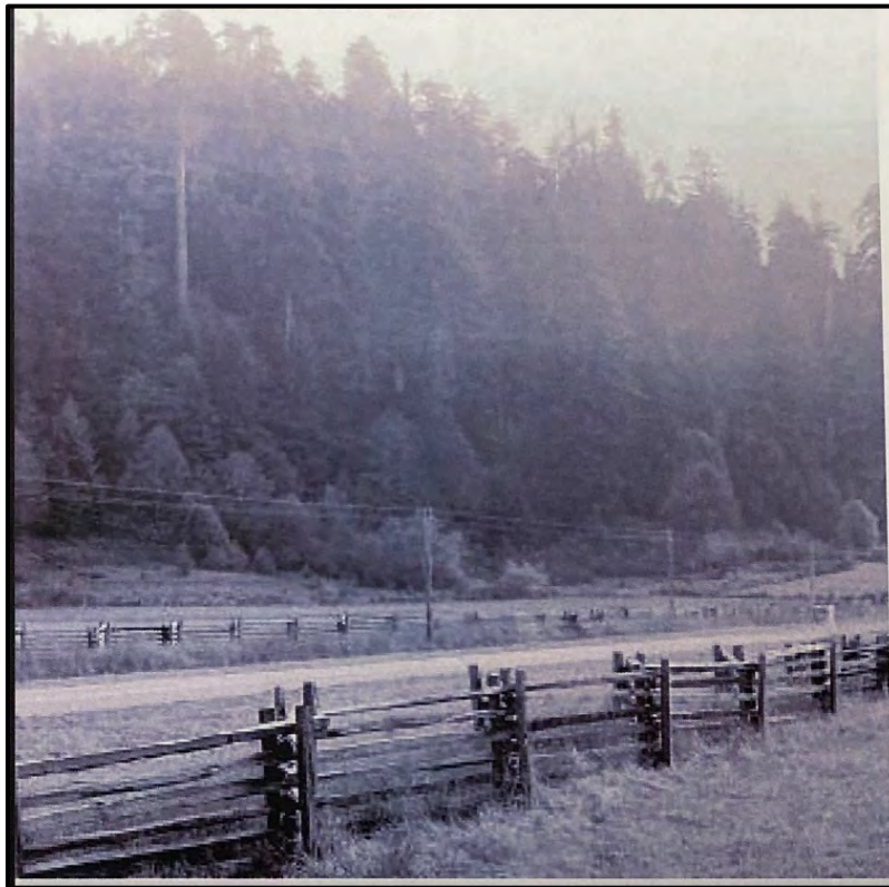
Figure 11. Split rail fence added by CCC along both sides of the Redwood Highway, April 1936. Source: California State Parks, North Coast Redwoods District Collection.
