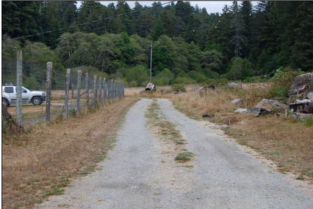
Figure 40. Circulation Features. Road to water treatment plant buildings and structures.
