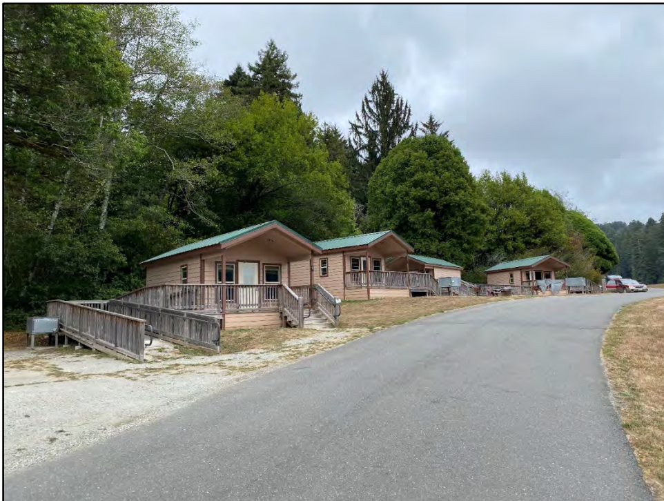
Figure 65. Buildings and Structures. Modern Seasonal Cabins (Cabins 1 through 4) near Campground.
