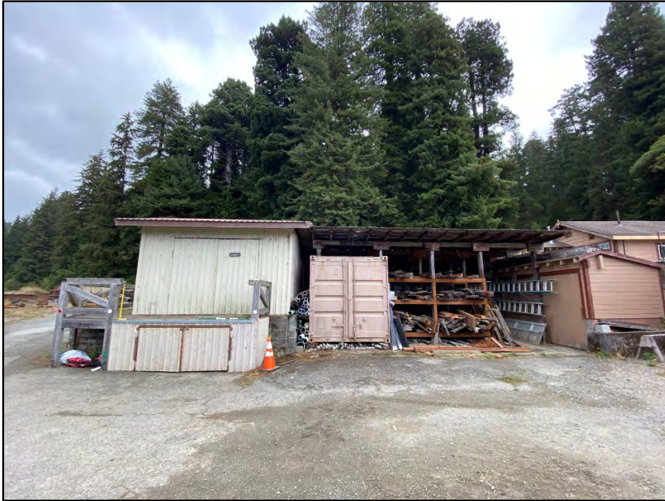
Figure 70. Buildings and Structures. Miscellaneous Storage and Shops cluster in the group of public works facilities that are east of the Boyes House.
