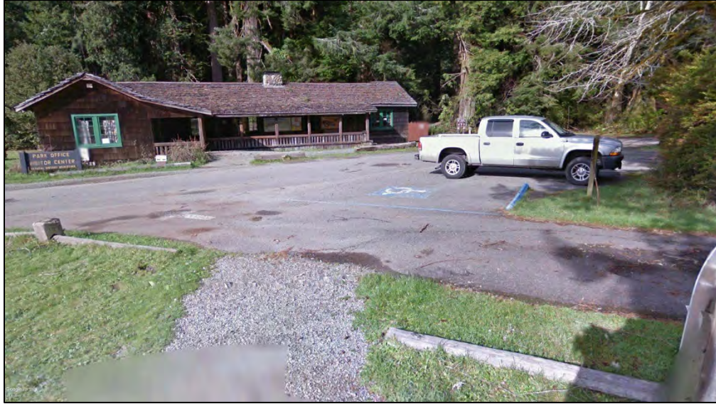
Figure 30. Circulation Features. This configuration for the Visitors Center parking lot dates from the 1960s.
