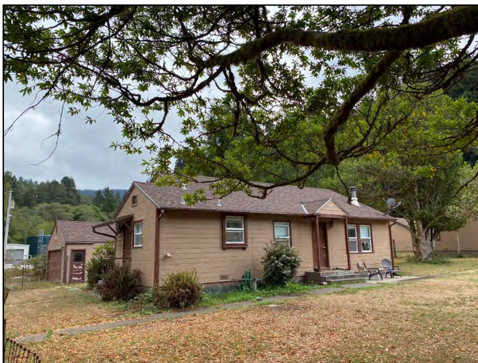
Figure 59. Buildings and Structures. Staff Residence #2 and Garage (1948).
