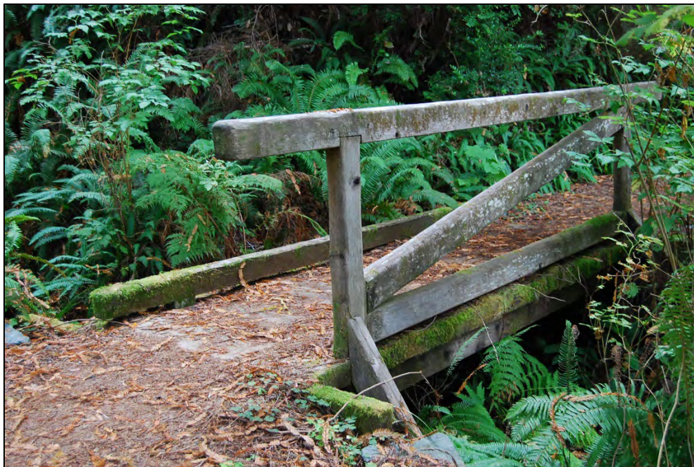
Figure 50. Circulation Features. Representative example of the bridges along Elk Prairie Trail. These bridges were rebuilt in late 1990s.
