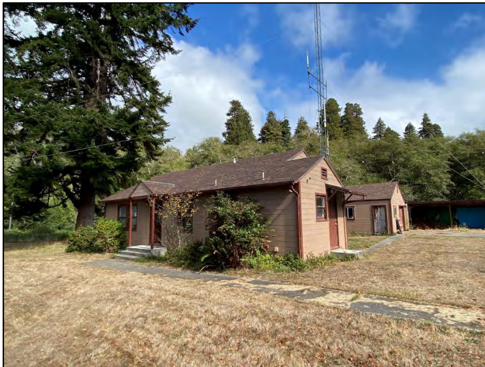
Figure 58. Buildings and Structures. Staff Residence #3 and Garage (1948).
