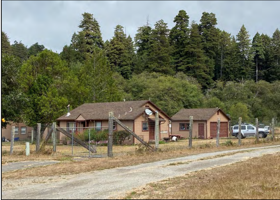
Figure 60. Buildings and Structures. Staff Residence #4 and Garage (1949).
