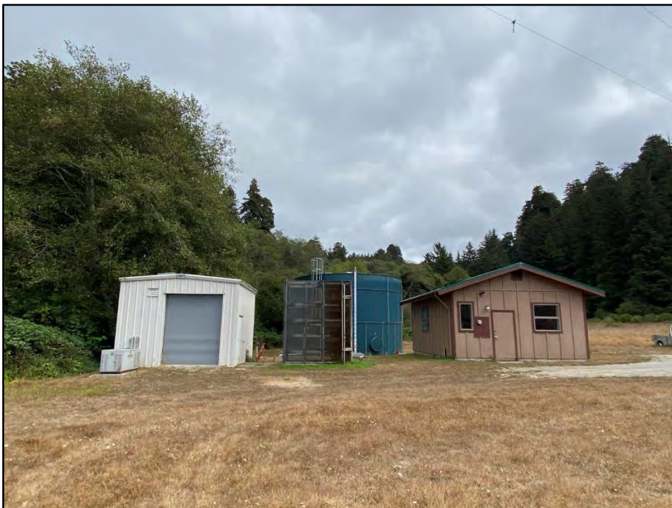
Figure 69. Buildings and Structures. Water Treatment Plant located behind Staff Residences, consisting of pump and water treatment houses, riveted steel tank, and aeration tower.
