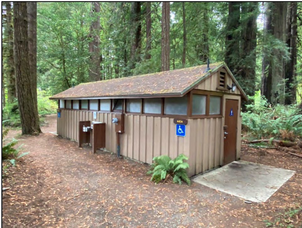
Figure 55. Buildings and Structures. Comfort Building at Revelation Trail (1948).
