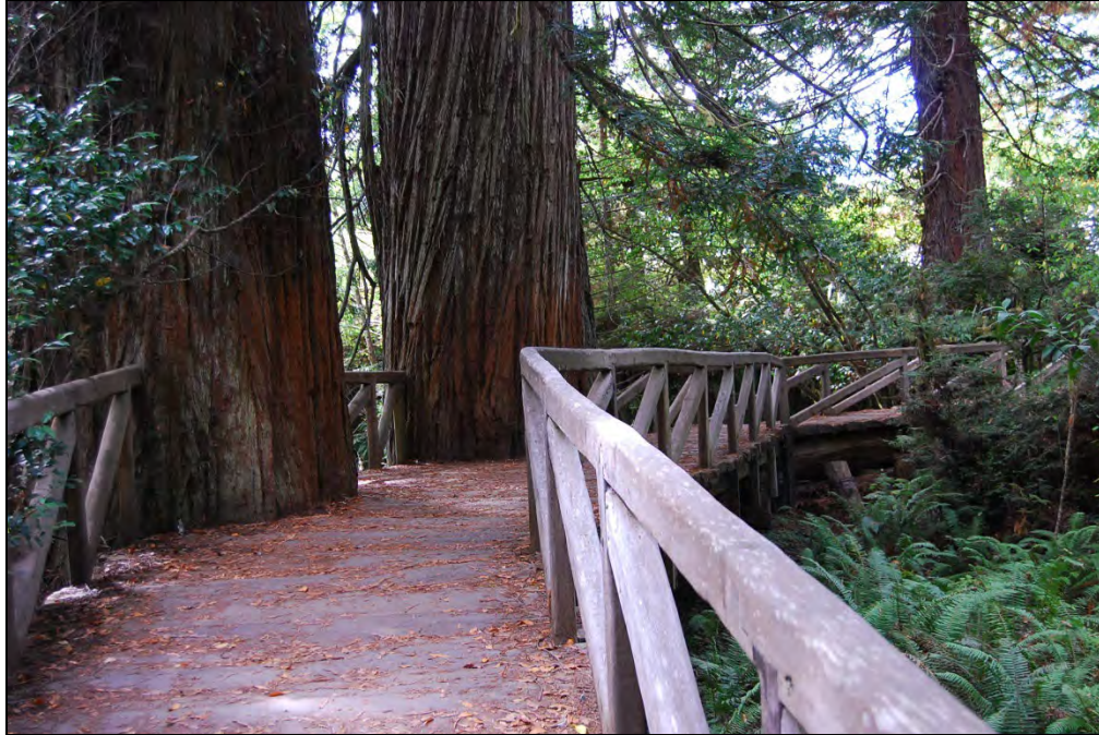
Figure 49. Circulation Features. Bridge over Prairie Creek. A bridge was built in this general location by the CCC in the mid-1930s. The current bridge and its design date from 1982; the bridge was further modified in the early 2000s.
