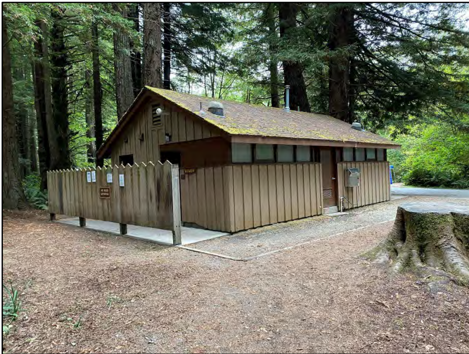
Figure 57. Buildings and Structures. Combination Building #3 (1949) at the Campground.
