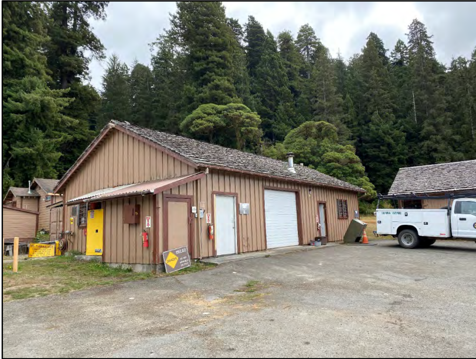
Figure 62. Buildings and Structures. Shop Building (1948) in the group of public works facilities that are east of the Boyes House.
