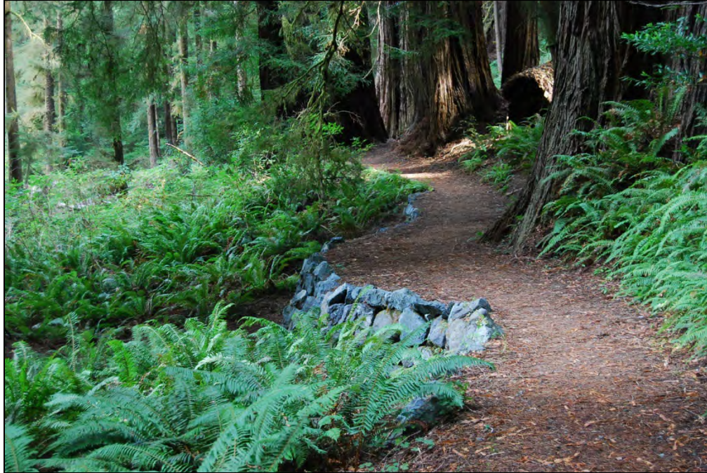
Figure 46. Circulation Features. Example of one of the retaining walls added to Elk Prairie Trail as part of rehabilitation project in the late 1990s.
