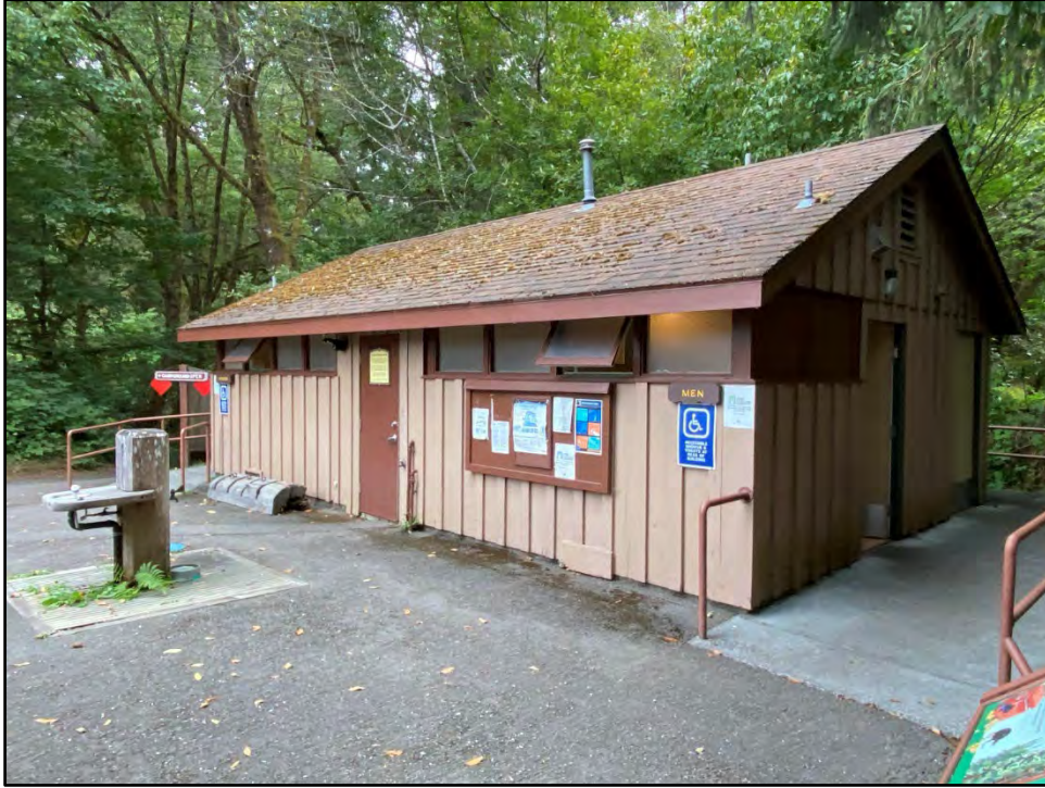
Figure 56. Buildings and Structures. Combination Building #2 (1949) at the Campground.
