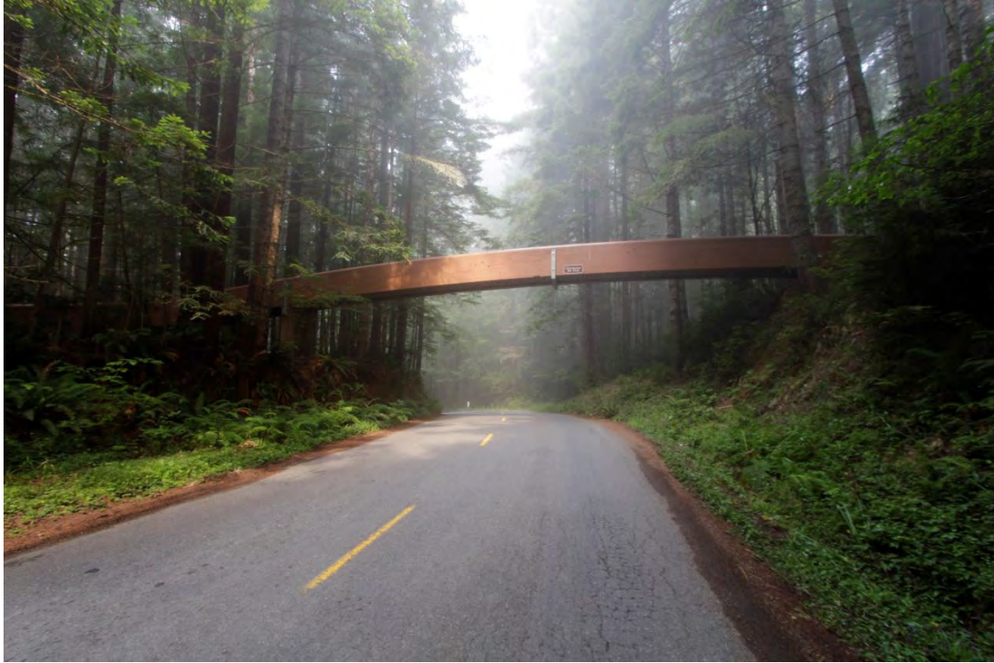
Figure 43. View of pedestrian bridge looking west from the current Bald Hills Road. [NPS 2018.]
