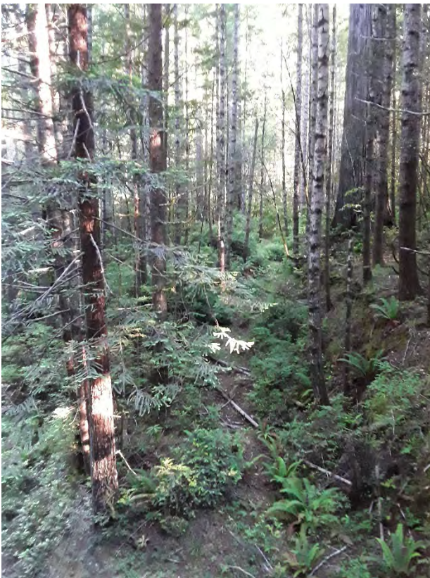
Figure 39. View from the pedestrian bridge looking down onto the former road alignment. The former alignment of Bald Hills Road was the original entrance to the grove. Today, the cutbanks can still be seen to the right, but are vegetated. [NPS 2021.]
