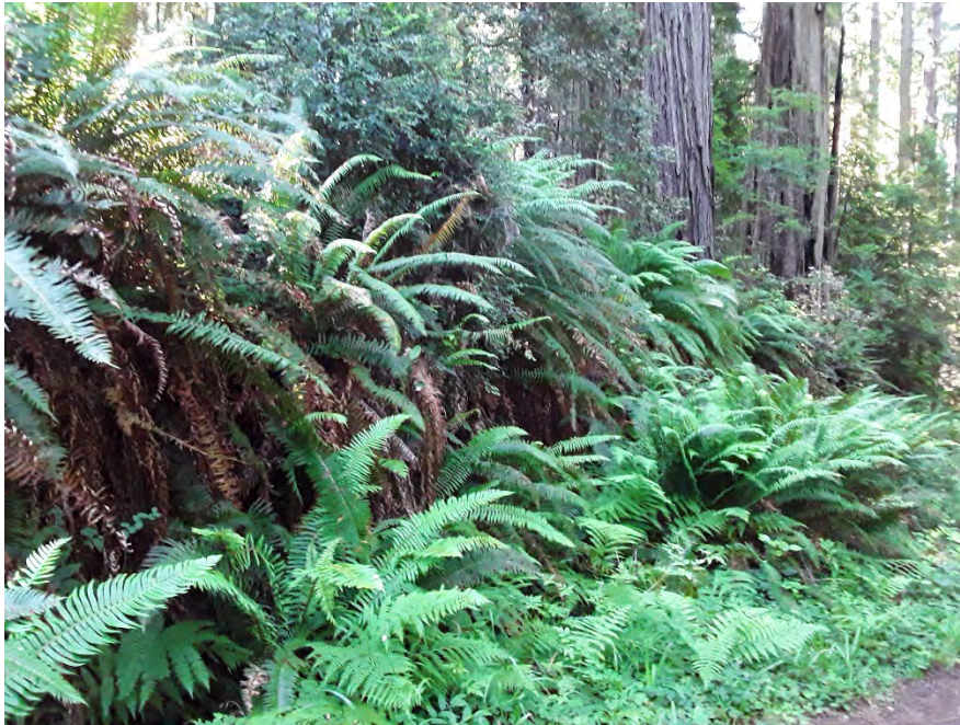
Figure 40. Example of a cut bank along Berry Glen Trail. [NPS 2021.]
