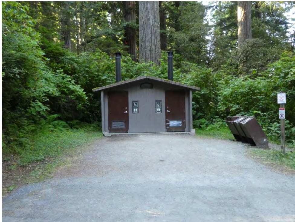
Figure 41. Concrete comfort station with two vault toilet restroom cells located on the south side of the parking lot. [NPS 2018.]
