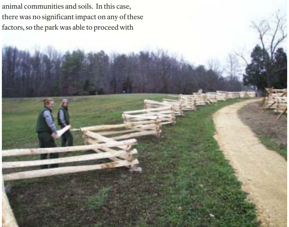
Beverly Bruce and Alisa Clark build worm fencing to mark the Watt House farm holdings on the Gaines' Mill battlefield unit of Richmond National Battlefield Park.
