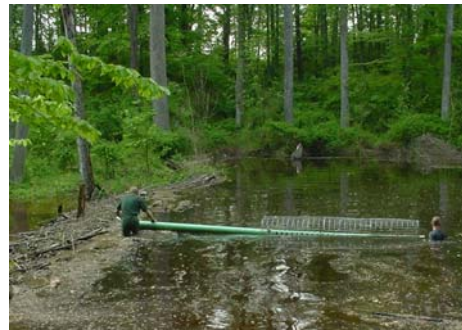
Left: Resource protection rangers Tim Mauch and Larry Smith place the "beaver baffle" on the dam at Boatswain Creek. Right: The baffle is successfully in place and draining the pond.
