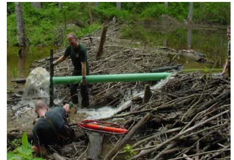
Left: Resource protection rangers Tim Mauch and Larry Smith place the "beaver baffle" on the dam at Boatswain Creek. Right: The baffle is successfully in place and draining the pond.
