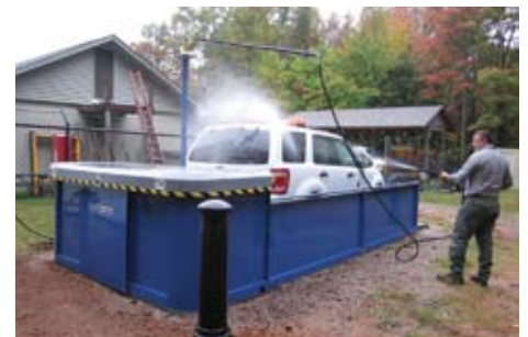
The parks' new eco-friendly wash bay recycles water and prevents chemicals and oil washed from the vehicles from entering the local watershed.
