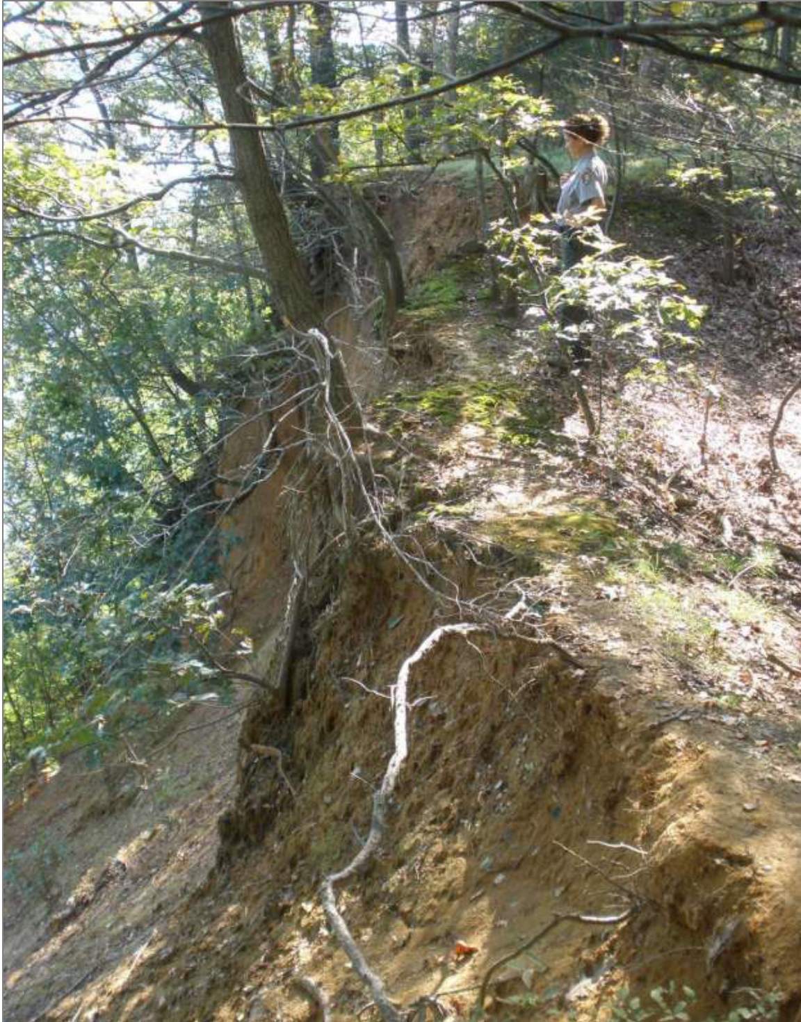
Figure 22. Photograph of near-vertical slopes at Drewry's Bluff. Failure and slumping in these steep areas are inevitable, and the bluff is inherently unstable. As slumping proceeds, the edge of the bluff will migrate some distance inland and the slope will eventually reach a new, temporary equilibrium. The material exposed on the face of the bluff is predominantly sand, gravel, and some clay layers in the Bacons Castle Formation (Qbc). Photograph is an unnumbered figure from Martin (2011).
