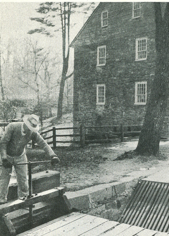
Regulating the flow of water in the mill race
