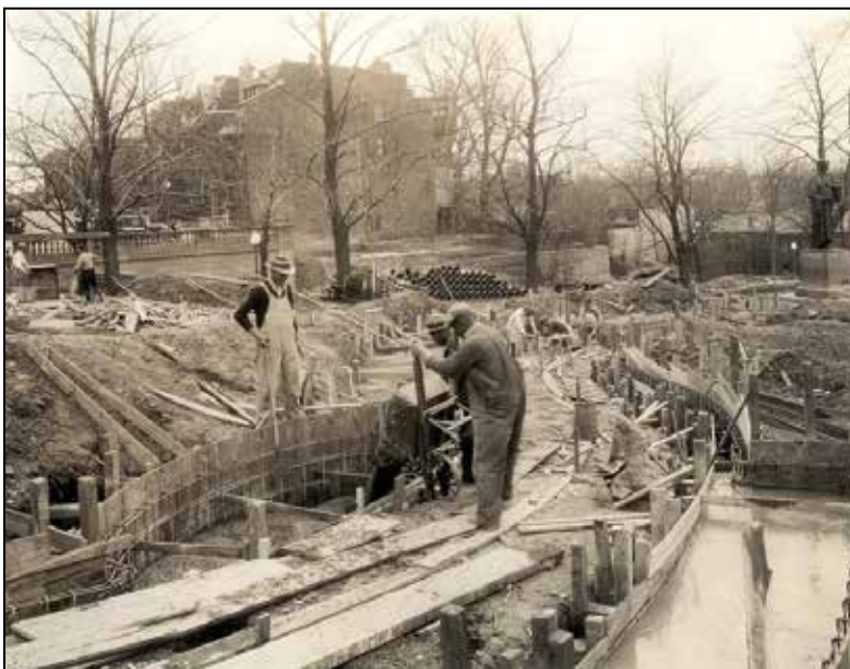
Figure 24: African American laborers creating a walkway to the Dante statue in Meridian Hill Park (National Park Service)
