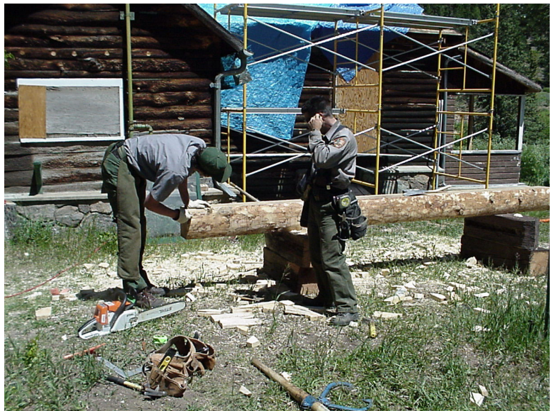
Park staff cut logs to repair a building at McGraw Ranch. (NPS-RMNP photo)
