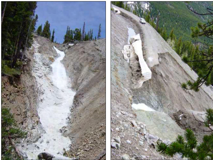
The failure of Grand River Ditch in 2003 resulted in erosion and sedimentation and contributed to the degraded condition of wetlands in Rocky Mountain NP.
