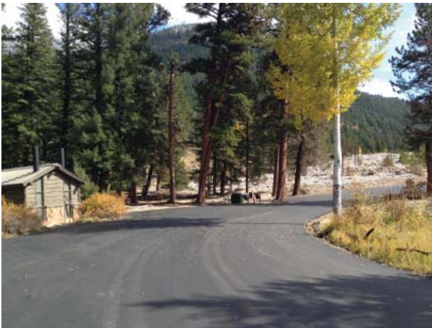
New pavement at West Alluvial parking lot. NPS Photo
