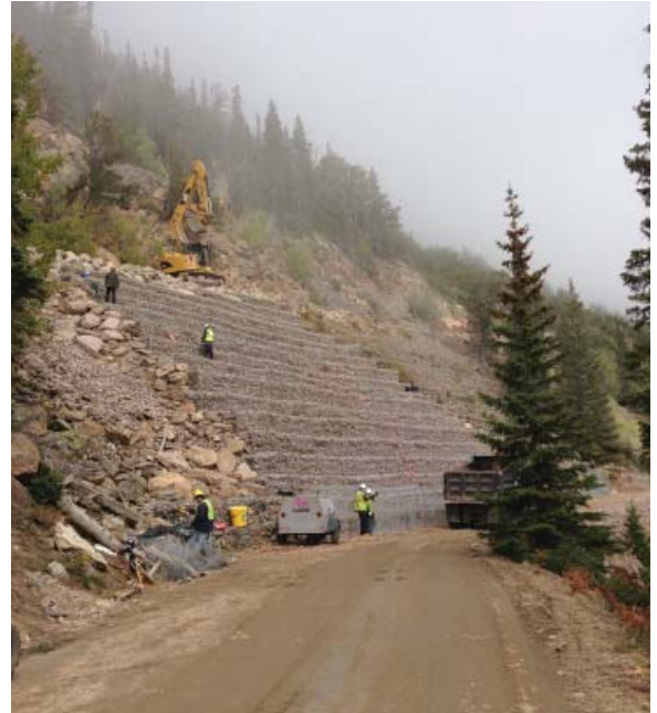
Installing gabions on Old Fall River Road. NPS Photo
