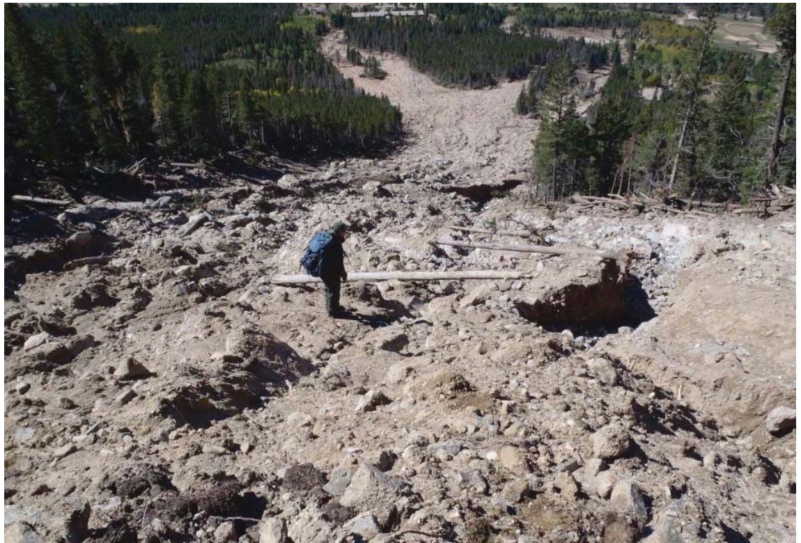
Damage to the Twin Sisters Trail from the September 2013 Flood
