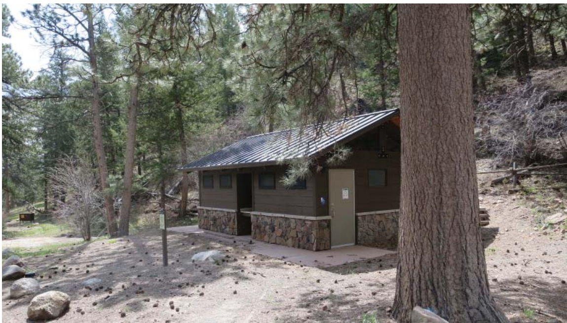
New accessible comfort station at Aspenglen Campground.
