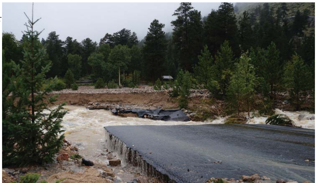
Endovalley Road looking west-bound after this section of the road was destroyed by the flood. NPS Photo
