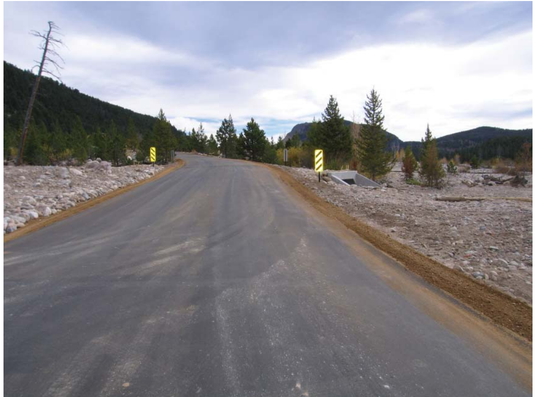
Endovalley Road looking east-bound, showing post-flood road repairs. NPS Photo
