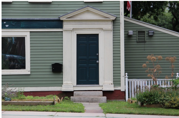
Exposed portions of foundation at north elevation.
