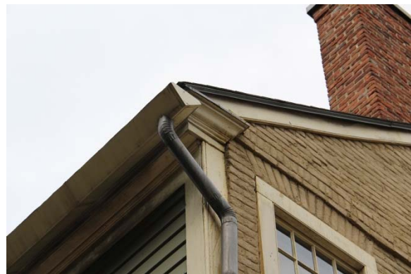
View of similar detail at southwest corner of house.
