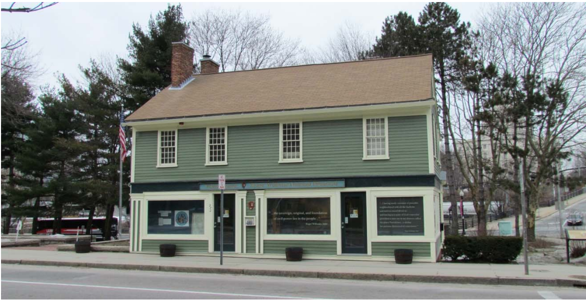
East Elevation at North Main Street. March 2015.
