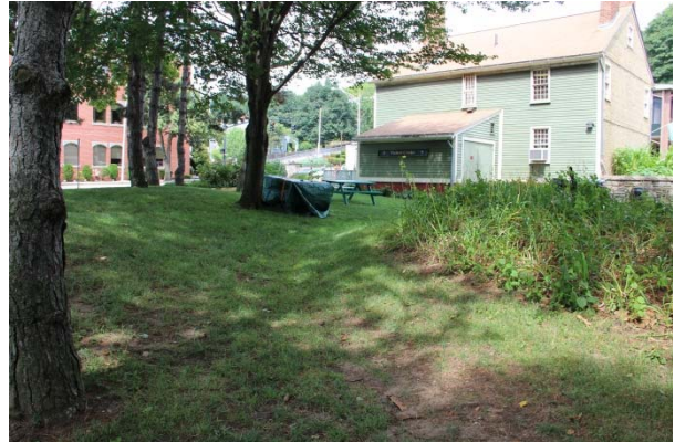
Drainage swale on west side of property directs site drainage away from generally elevated building site through a drainage swale incorporated into the site topography.
