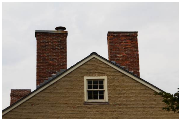
B10: Capped and sealed chimneys at south gable elevation.
