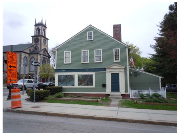
Positive drainage along Smith Street elevation and in front yard area.
