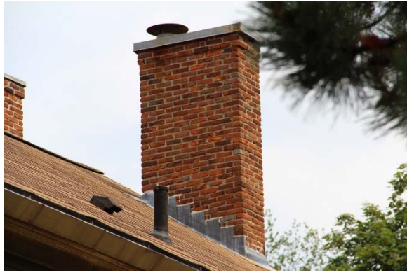
CH01 from the north
