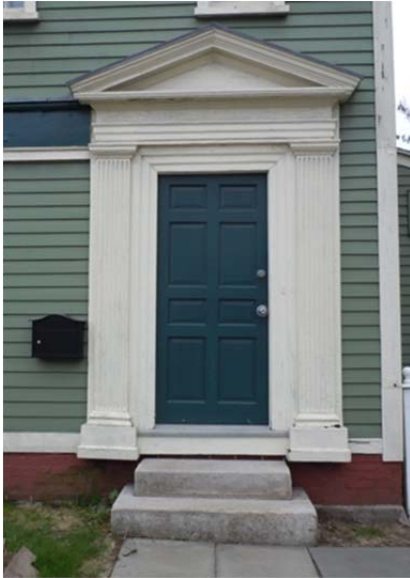
North elevation door with historic door surround; D103 is a modern panel door.
