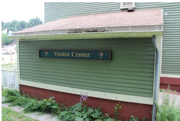
Single gutter run at shed with downspout.
