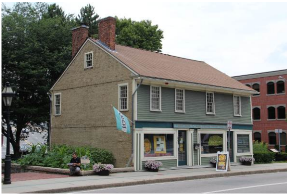
Overview of south brick gable end and east elevation illustrates several of the secondary features and trim components.
