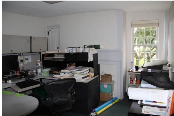
2 nd floor southwest chamber (office) with corner closet, fireplace over mantle and exposed corner post (painted gray) along brick south gable wall; W206 in corner.
