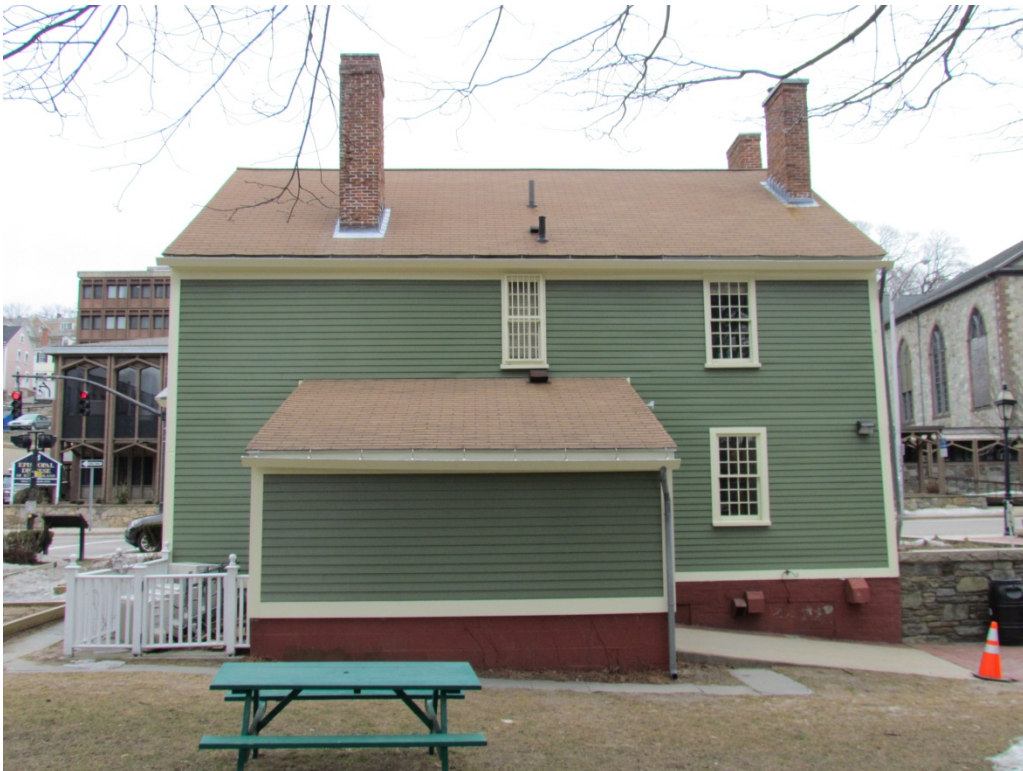
West elevation with Maintenance Shed Addition. March 2015.
