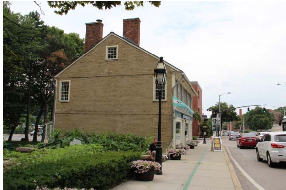
General slope of sidewalk is towards the south elevation of the house along North Main Street.
