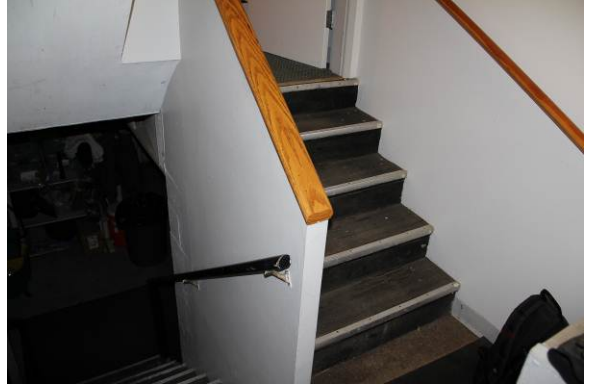
Non fire rated enclosure between basement and first floor.
