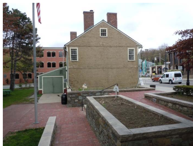
Positive drainage at pedestrian pathways to front entrance.
