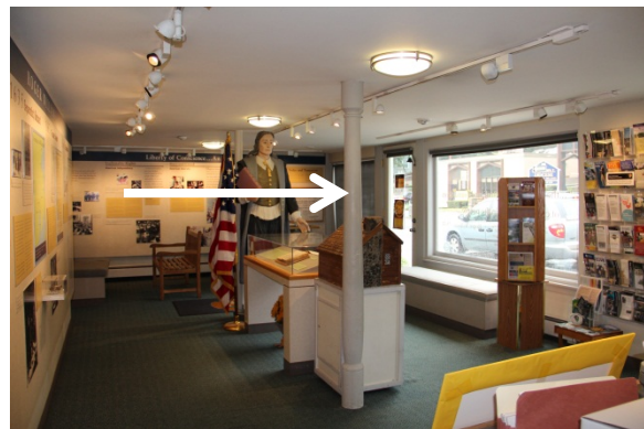
19 th C turned post is primary structural support in building frame.
