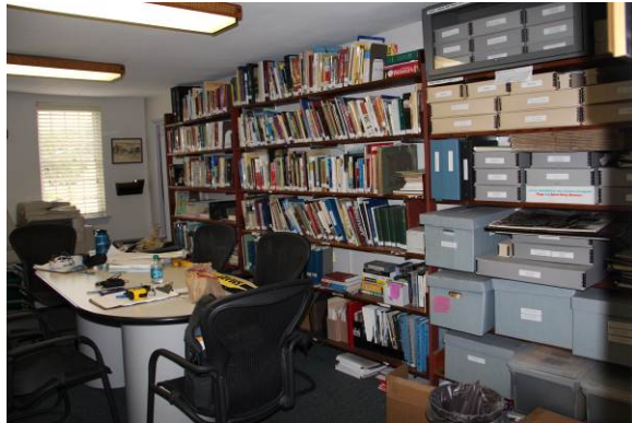
B10: Possible over-stressing of historic post and beam structure due to overloading of interior spaces.
