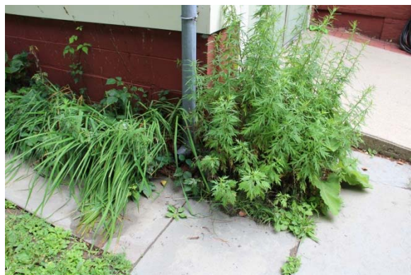
Downspout daylights at base of building.
