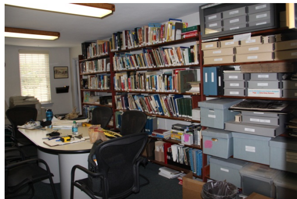
Possible over-loaded conditions at 2 nd floor – all heavy loads are placed around perimeter of room where structure is usually located lessening the chances of structural failure.
