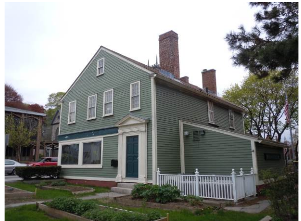
North and west elevations also carry several of the character-defining features mentioned above.
