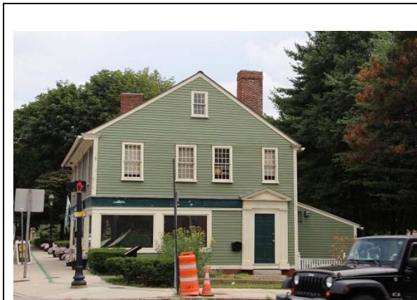
North Elevation at Smith Street, July 2014.
