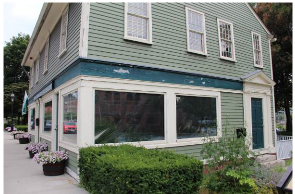
Condition of exterior painted surfaces, July 2014.
