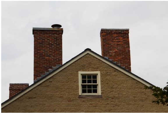
Capped and sealed chimneys at south gable elevation.
