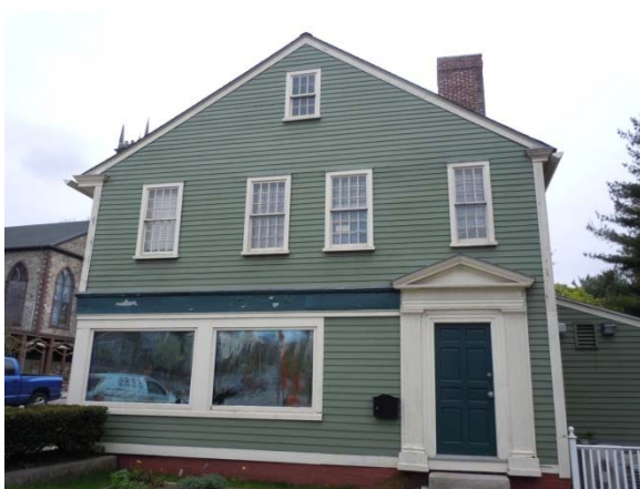
North elevation with exterior clapboarding in good condition.
