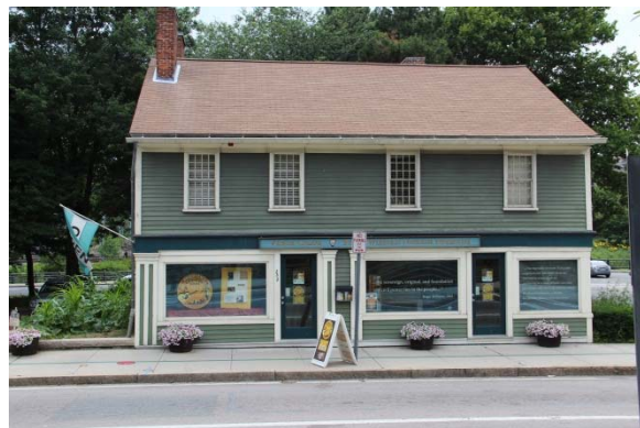
East Elevation at North Main Street, July 2014.
