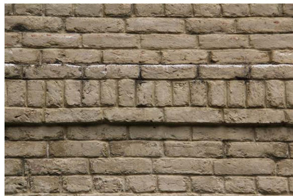
Detail of projecting triple course brick water table on south elevation.
