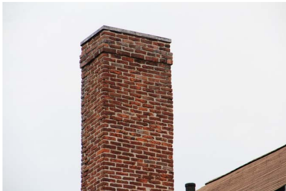
CH03 from the south
