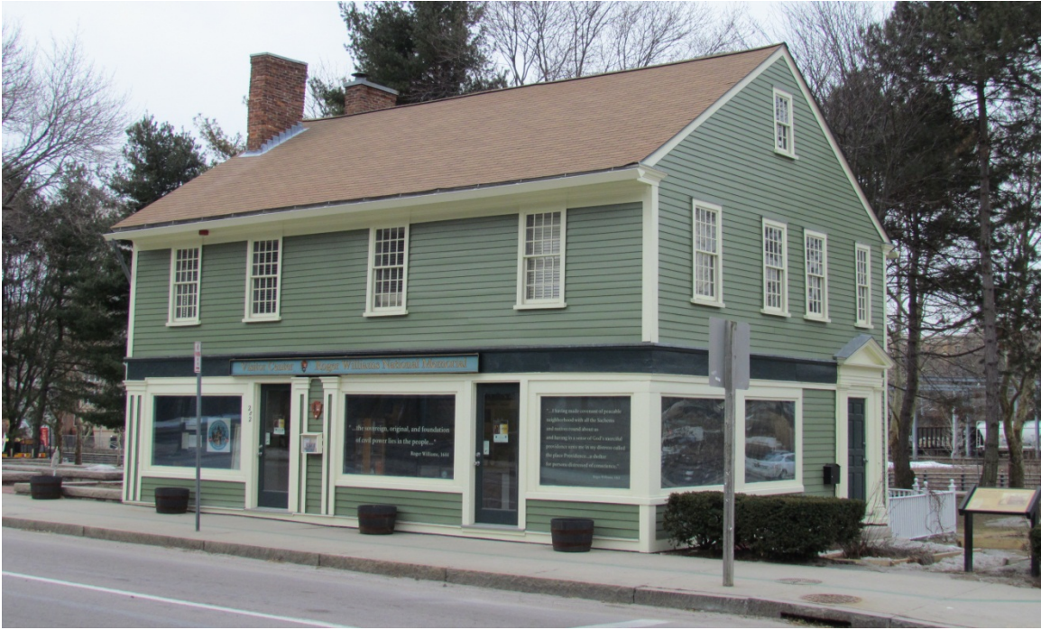
Northeast elevations, corner of Main and Smith Streets. March 2015.
