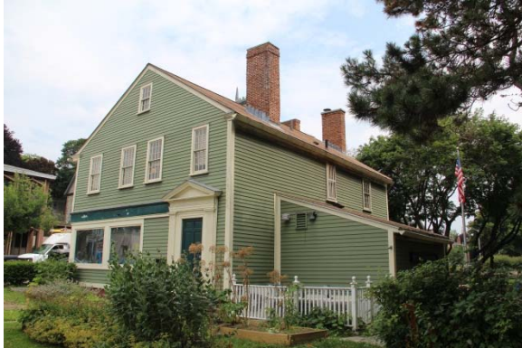
Fenced area to west of primary architectural feature of north elevation contains condensing units for Mitsubishi split system.
