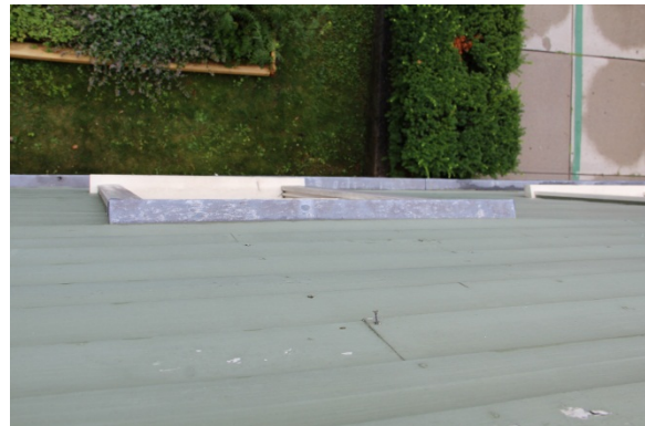
View of lead-coated copper window flashing as seen from attic window.
