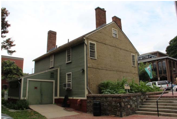
General slope of site is away from southwest corner of house.
