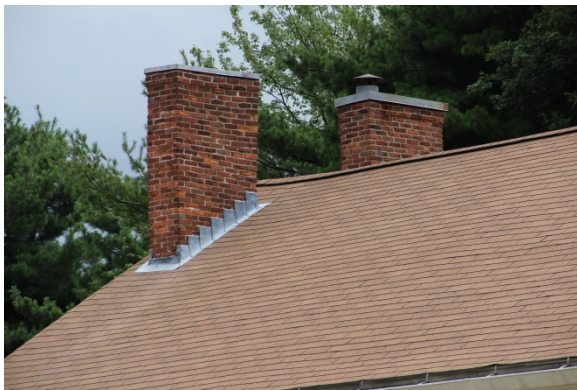
South gable chimneys with caps as seen from the northeast.
