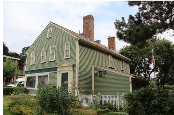
Interior chimney near the north end of the house on the west slope of the roof.
