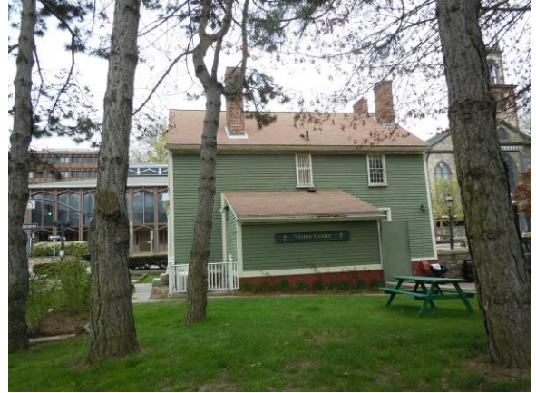
West Elevation from park grounds. Visual prominence of fiberglass shingle roof is inappropriate for a historic house representing the earliest settlement of Providence time period.
