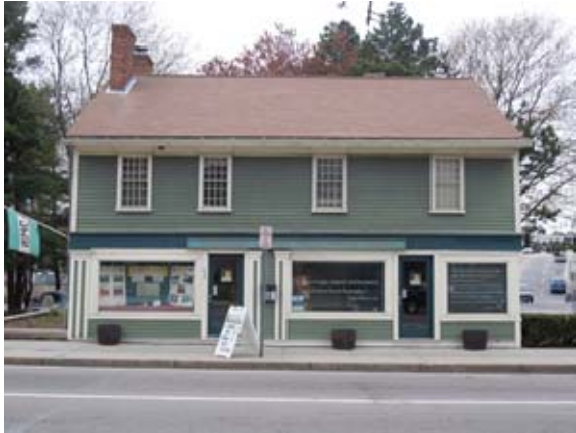
East Elevation at North Main Street. Fiberglass shingle roof lacks texture and color of traditional character-defining wood shingle roof.
