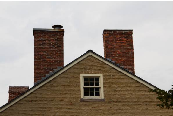
The twin south gable end chimneys are primary roof features on the gabled roof.
