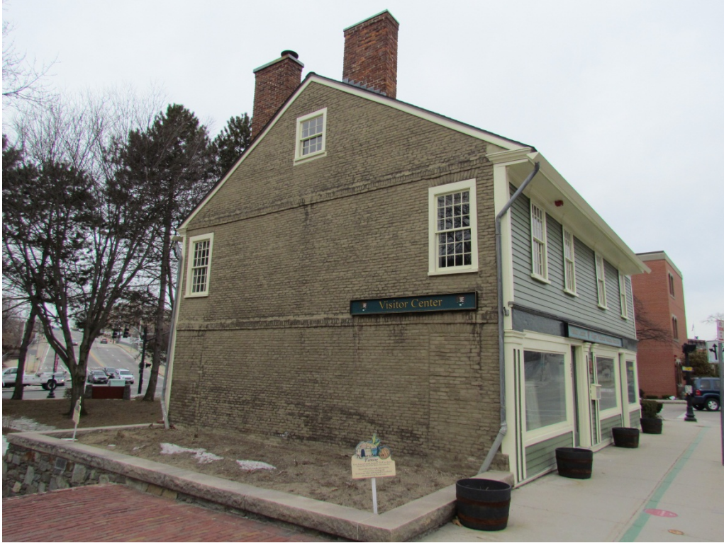
South and East elevations. March 2015.
