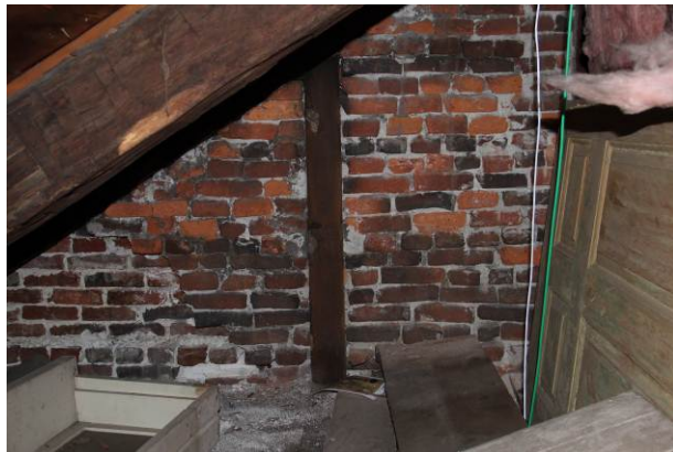
Unpainted (repaired) interior wall surface of south gable wall from attic.
