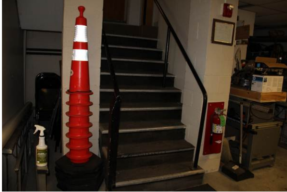
Open stair between floors; also functions as main egress from basement offices.
