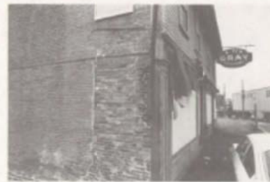
Illustration 71. Antram-Gray House: South Facade, East End.
