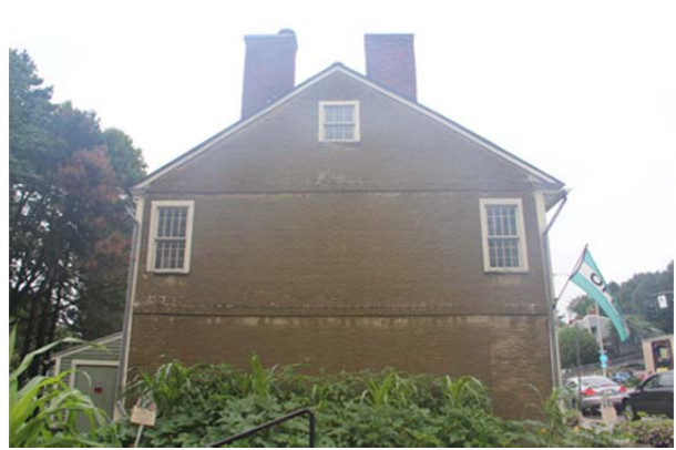
View of south gable end after rainstorm, note wetting pattern of brick; all water drains into planter bed at base of wall (where corn is growing).
