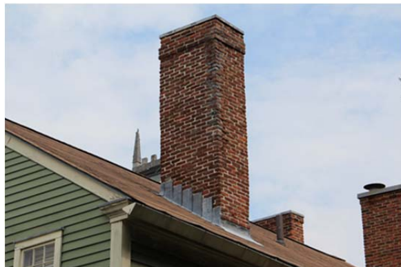
CH03 from the north
