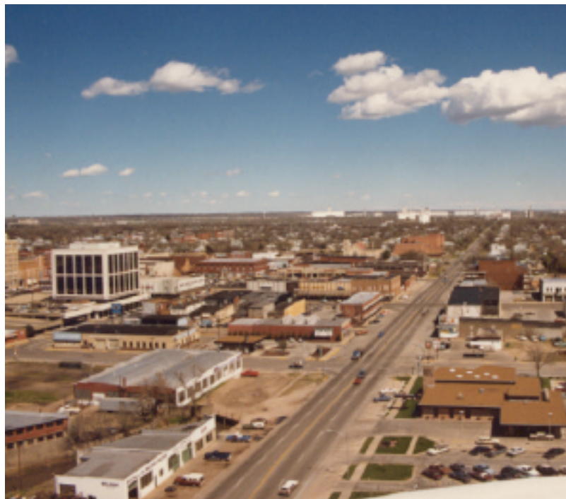
Avenue A in Hutchinson, Kansas before daylighting Cow Creek. This area frequently flooded during winter storms.
