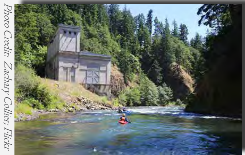
PacifiCorp Powerhouse seen from the river
