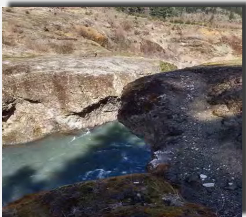
Site of the of Condit Dam
