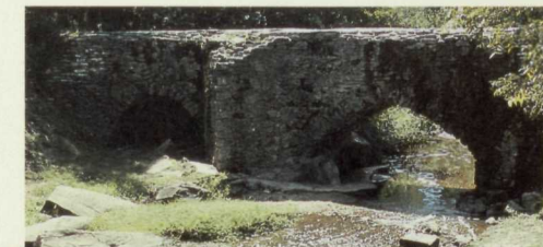
The arches of the two-centuries-old Espada Aqueduct.
