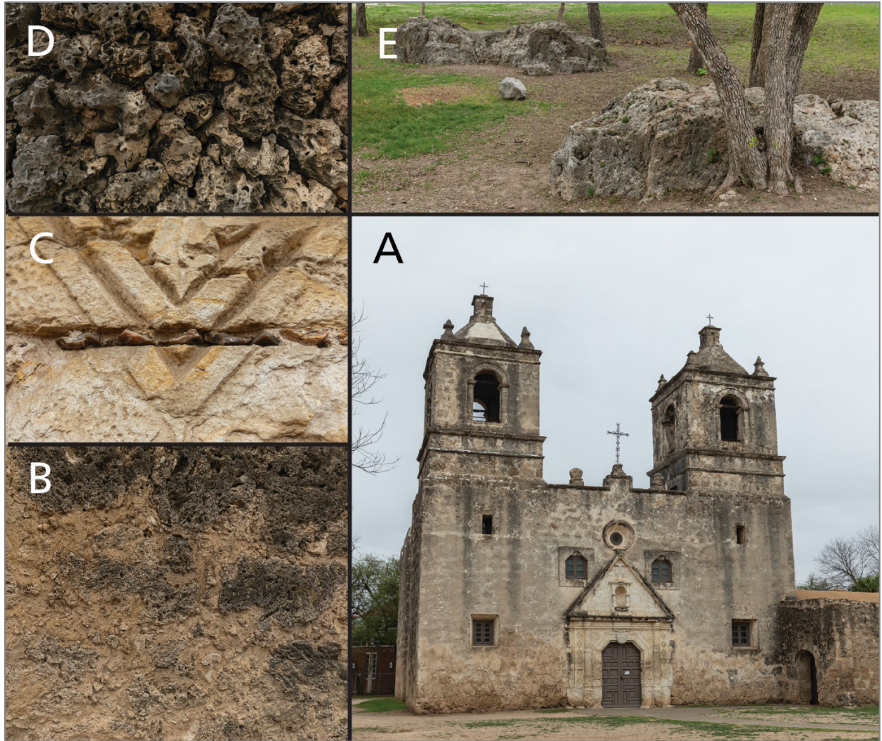
Figure 6. Photographs of Missions Concepción. A) The façade of Mission Concepción. B) A close-up photo of the texture of the remnant plaster covering the tufa used in construction of the mission. The plaster was also created using locally available geologic resources. C) A close-up photo of the Austin Limestone carved for the portico on the mission along with the decorative chert placed in chiseled-out lines. D) Texture of the Concepción tufa. E) The location of one of the historic quarries that was utilized during the construction of Mission Concepción. Photos by Matthew Harrington (Colorado State University).
