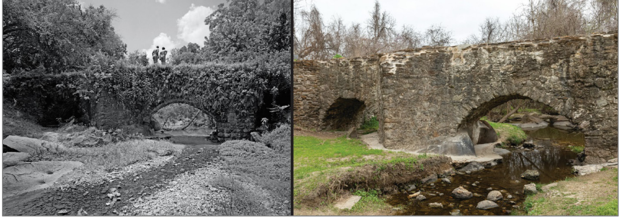
Figure 14. The Espada Aqueduct in 1936 and 2023. Originally constructed in the 1730s, the Espada Aqueduct is the oldest Spanish aqueduct in the United States. Although most of the missions have seen considerable change since their initial construction, the Espada Aqueduct has successfully survived over 275 years of floods, storms, and urban expansion. The first photo shows the Espada Aqueduct in 1936. The second photo shows the Espada Aqueduct as it looked in 2023. In both photos, Piedras Creek, which flows beneath the aqueduct, has a similar pattern of flowing under the right arch of the aqueduct. The first photo was taken by an unknown Historic American Buildings Survey photographer, courtesy of David Vekasy, NPS. The second photo was taken by Matthew Harrington (Colorado State University).
