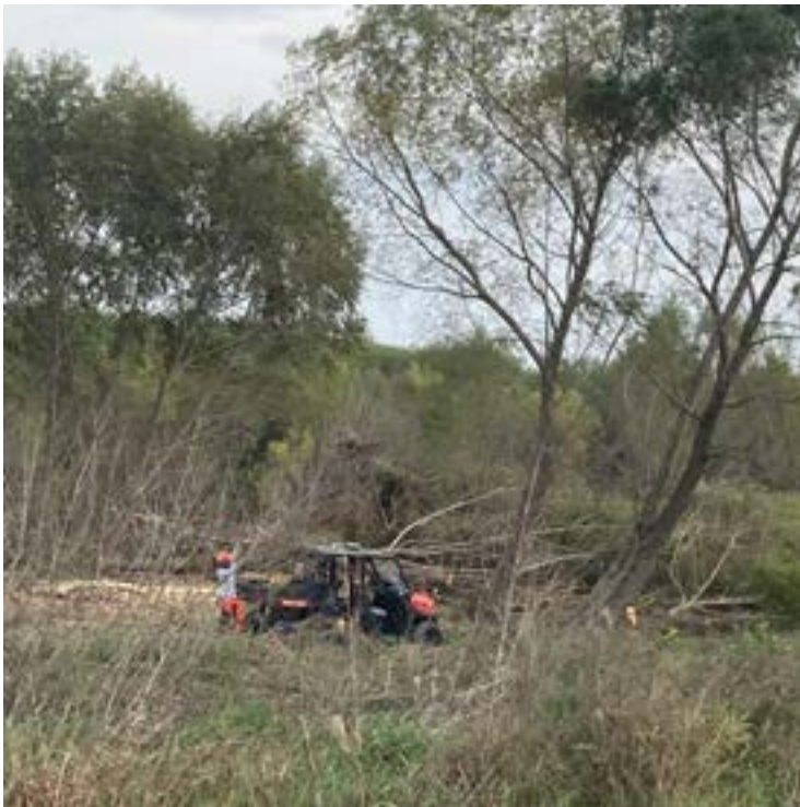
River Authority crews removing trees from the Mission Reach.
