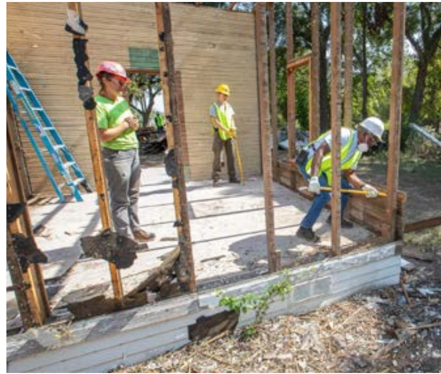
Crew in safety gear deconstructing an old home.
