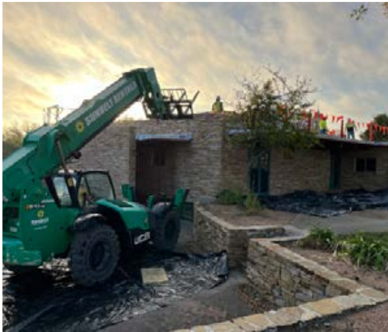
Rehabilitation work on the historic roof of the Harris House.
