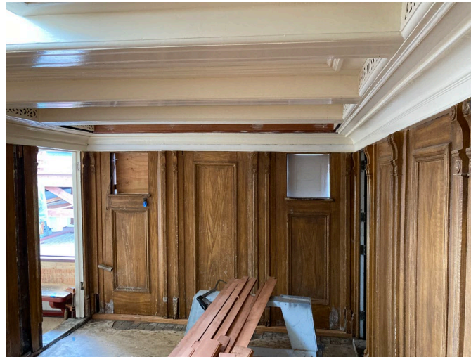
Photo 3: The deck houses are lighter wood framed construction and pose a potential moderate fire growth rate.
