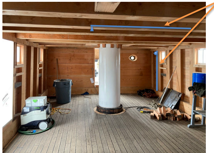
Photo 10: The water mist nozzles may be ceiling or wall mounted with tube integrated into wall fabric or surface mounted to minimize visual impact. The tube diameter for an individual nozzle will be 12 mm.
