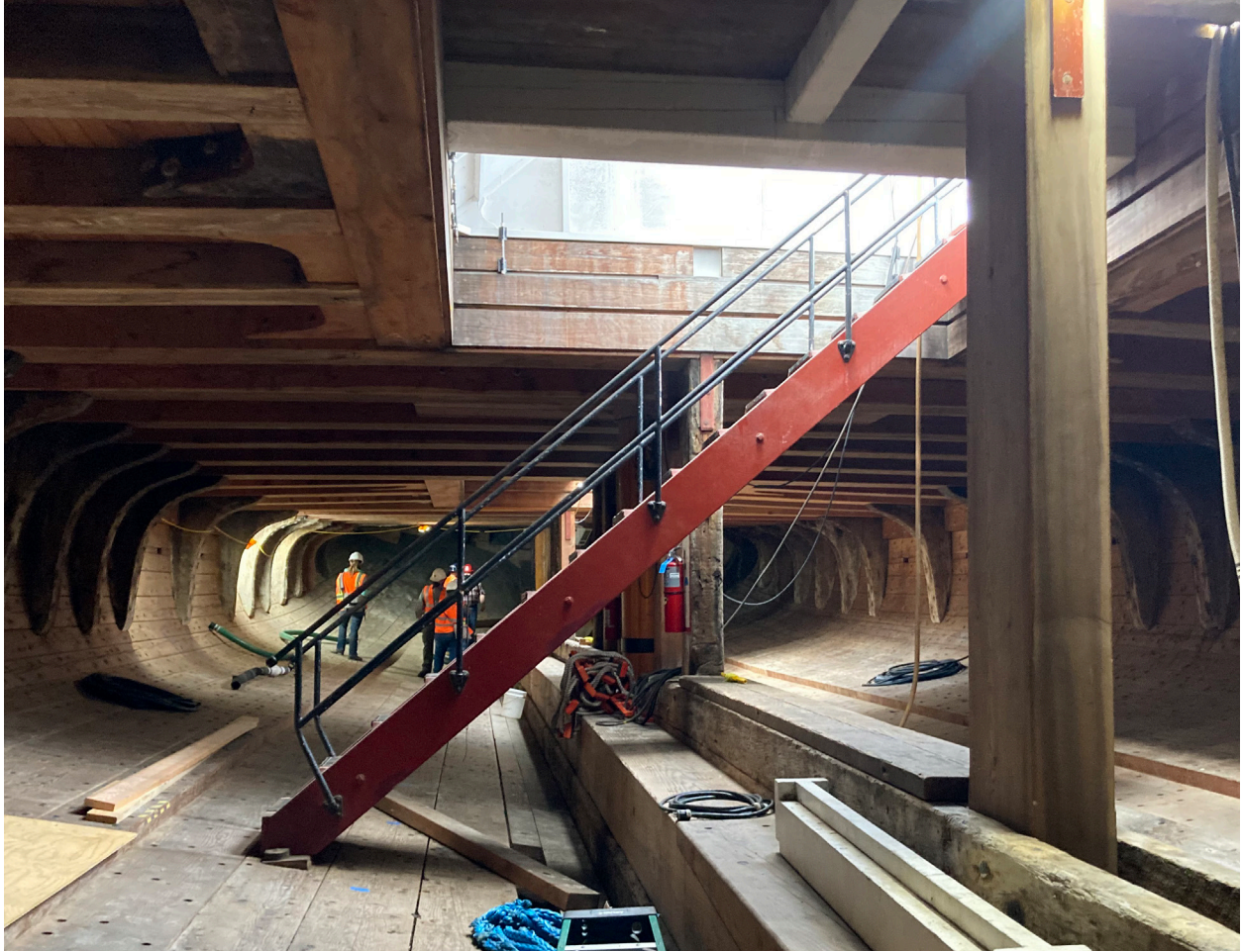
C.A. Thayer, view inside hold, 2020 (Architectural Resources Group).
