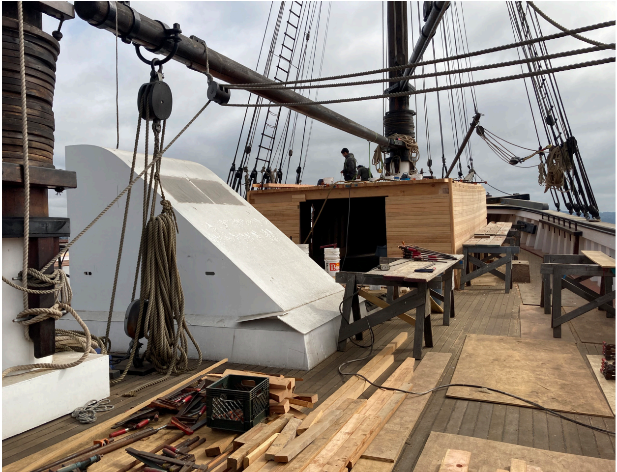
C.A. Thayer in dry dock, 2020 (Architectural Resources Group).
