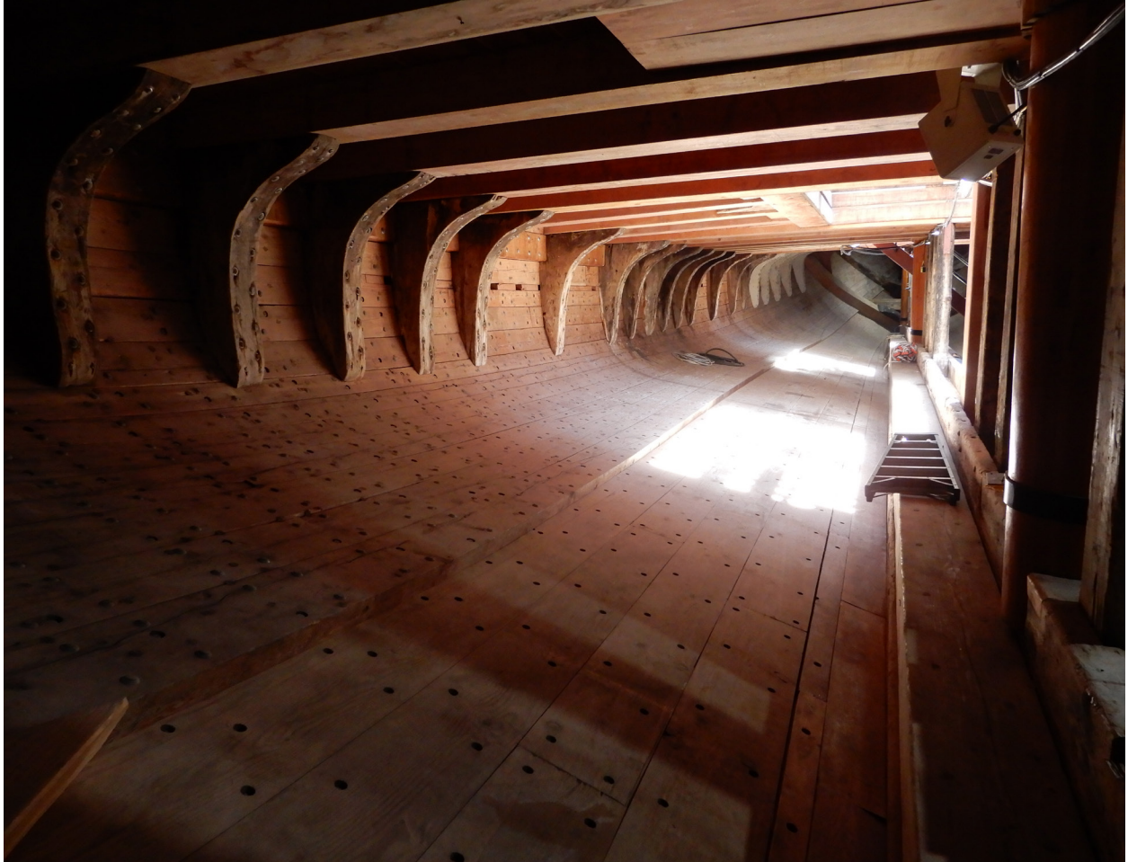
C.A. Thayer, view inside hold, 2021 (Architectural Resources Group).
