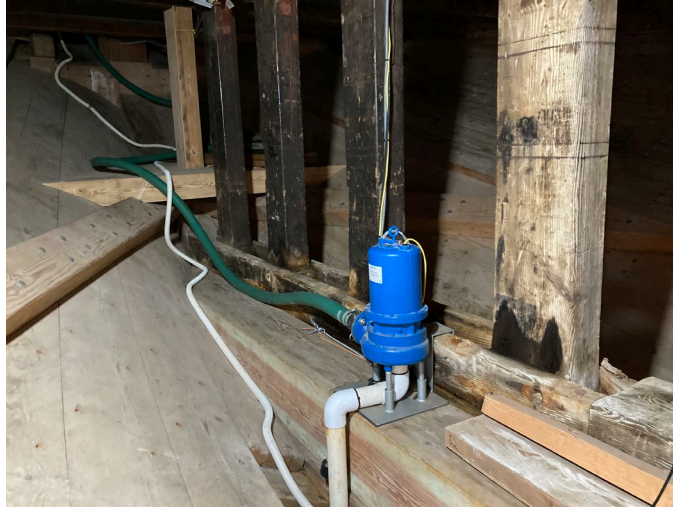
Photo 4: The bilge pump is one of the higher ignition threats but this hazard can be controlled by placing the pump in a metal cabinet to prevent the pump from contacting the wood elements.
