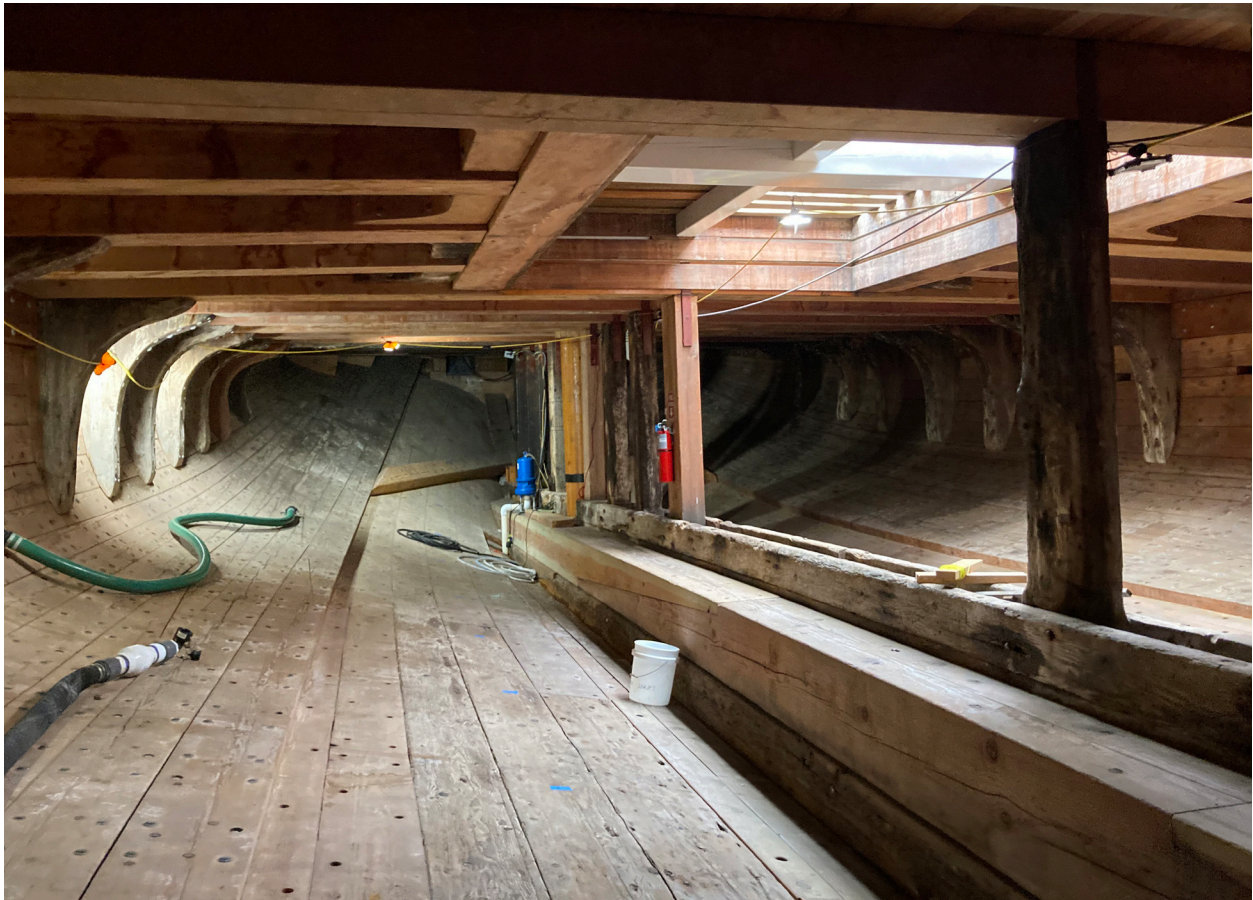
C.A. Thayer, view inside hold, 2020 (Architectural Resources Group).
