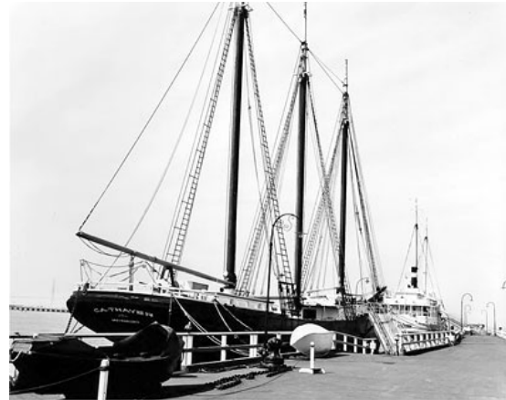
Figure 8. C. A. Thayer at the San Francisco Maritime State Historical Park at Hyde Street Pier, 1965. Source: National Register Nomination, 1966.
