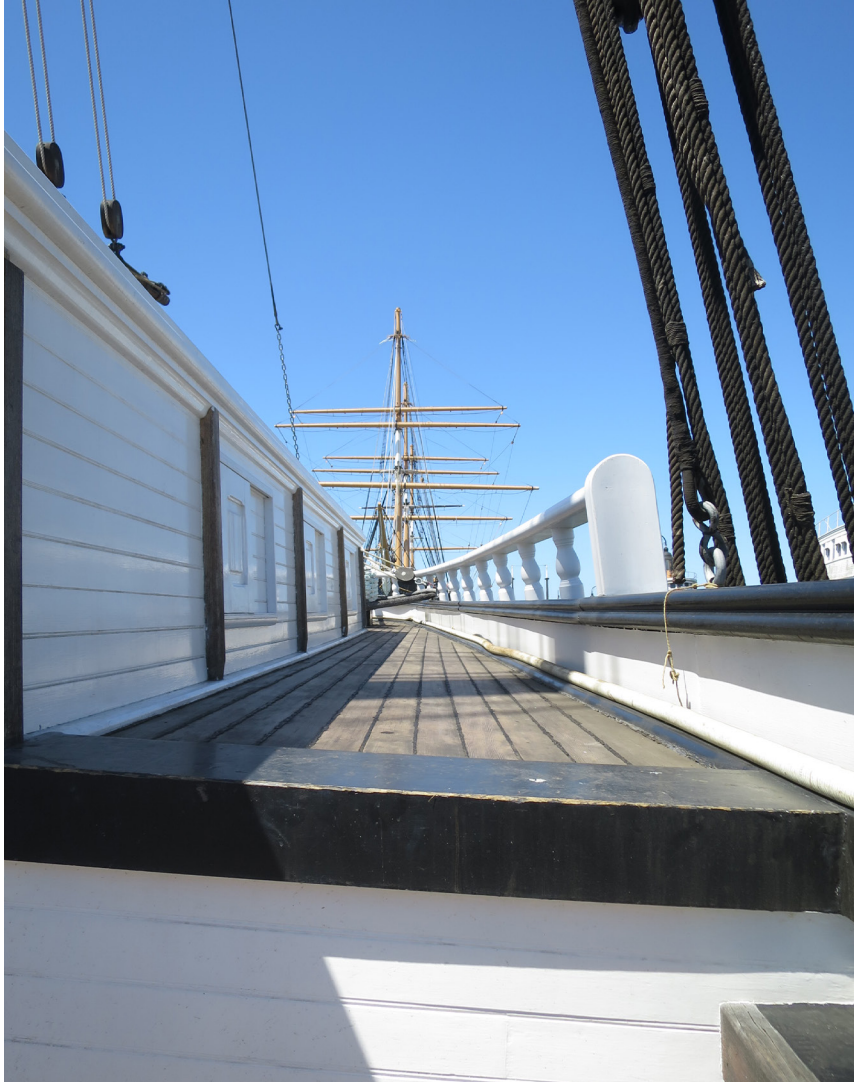
C.A. Thayer, view on poop deck, 2021 (Architectural Resources Group).
