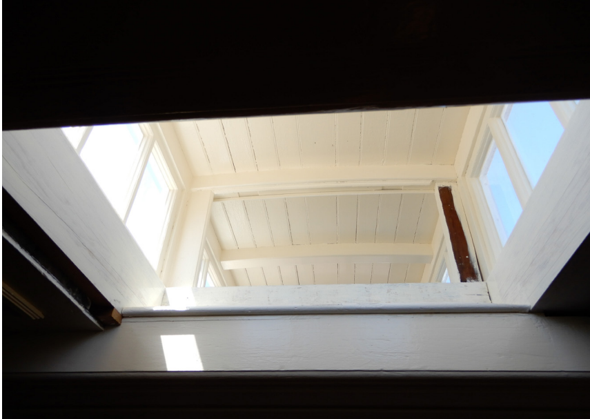
C.A. Thayer, view inside aft cabin, 2021 (Architectural Resources Group).
