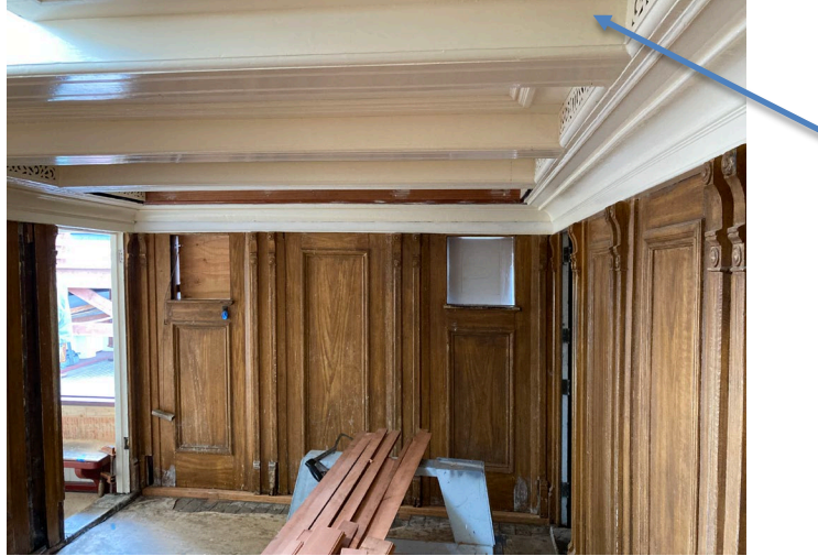
Photo 11: Mist nozzles apply water in a three dimensional mode which creates a cloud like spray. This allows greater flexibility than standard sprinklers. A nozzle integrated into the grates could cover the fire hazard within this entire deck house space.
