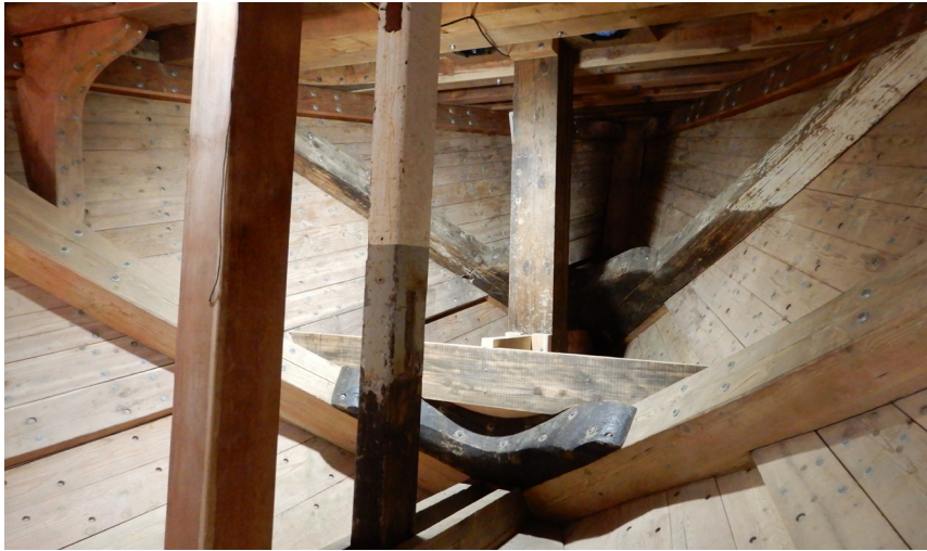
C.A. Thayer, view inside hold, 2021 (Architectural Resources Group).
